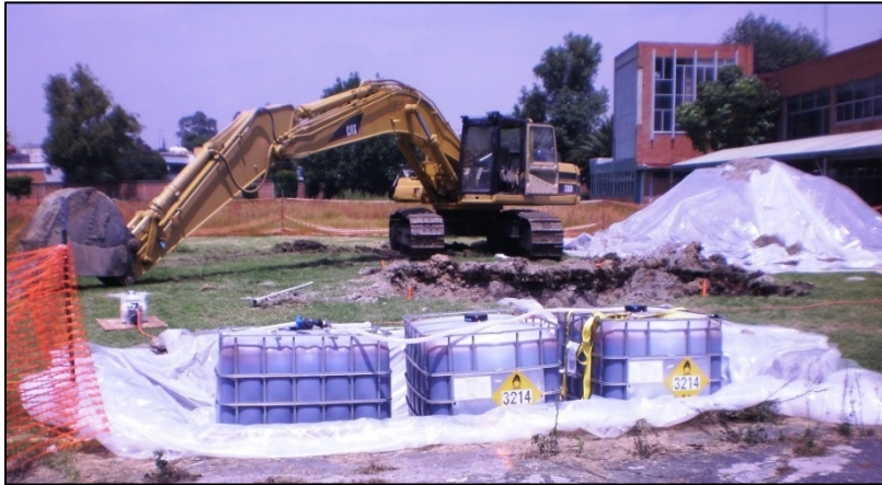
Photo: ISCO Soil Mixing
