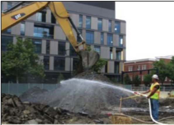
Photo: Vapor Suppression
