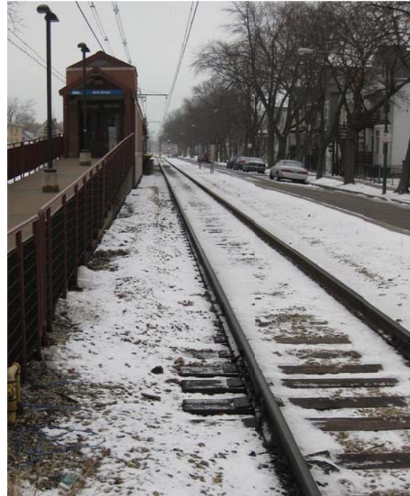
Figure 5-9: Metra Electric District South Chicago Branch Infrastructure and Track at 83rd Street Station
