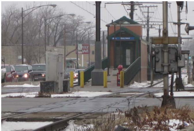
Figure 5-13: Metra Electric District South Chicago Branch Stony Island Station Entrance
