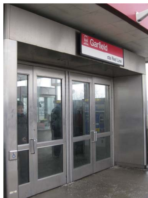
Figure 5-5: CTA Red Line Garfield Station Main Entrance
