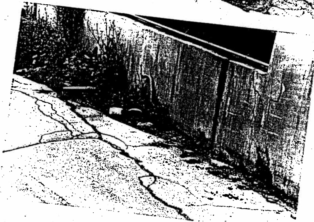
PHOTO S-13 Exterior or retaining wall.
