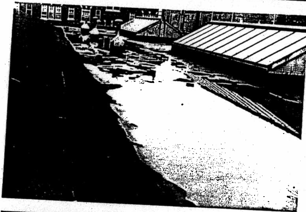
PHOTO A-5 Ponding water on roof and skylights.
