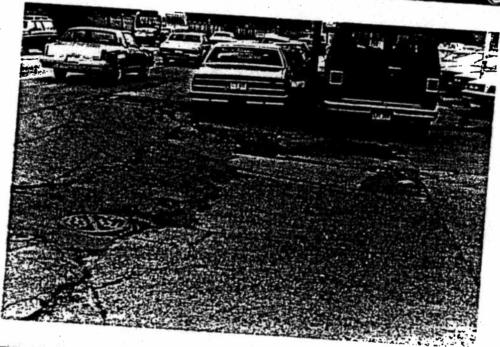
PHOTO C-2 Aged and deteriorated paving.
