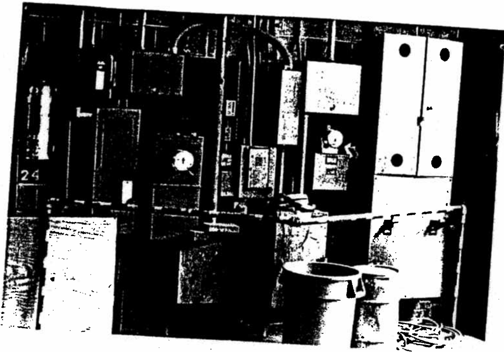
PHOTO E-2 Rusted out electrical service distribution for the west building.
