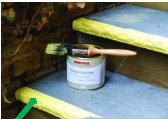
Bright Paint Makes Stairs Easy to See
