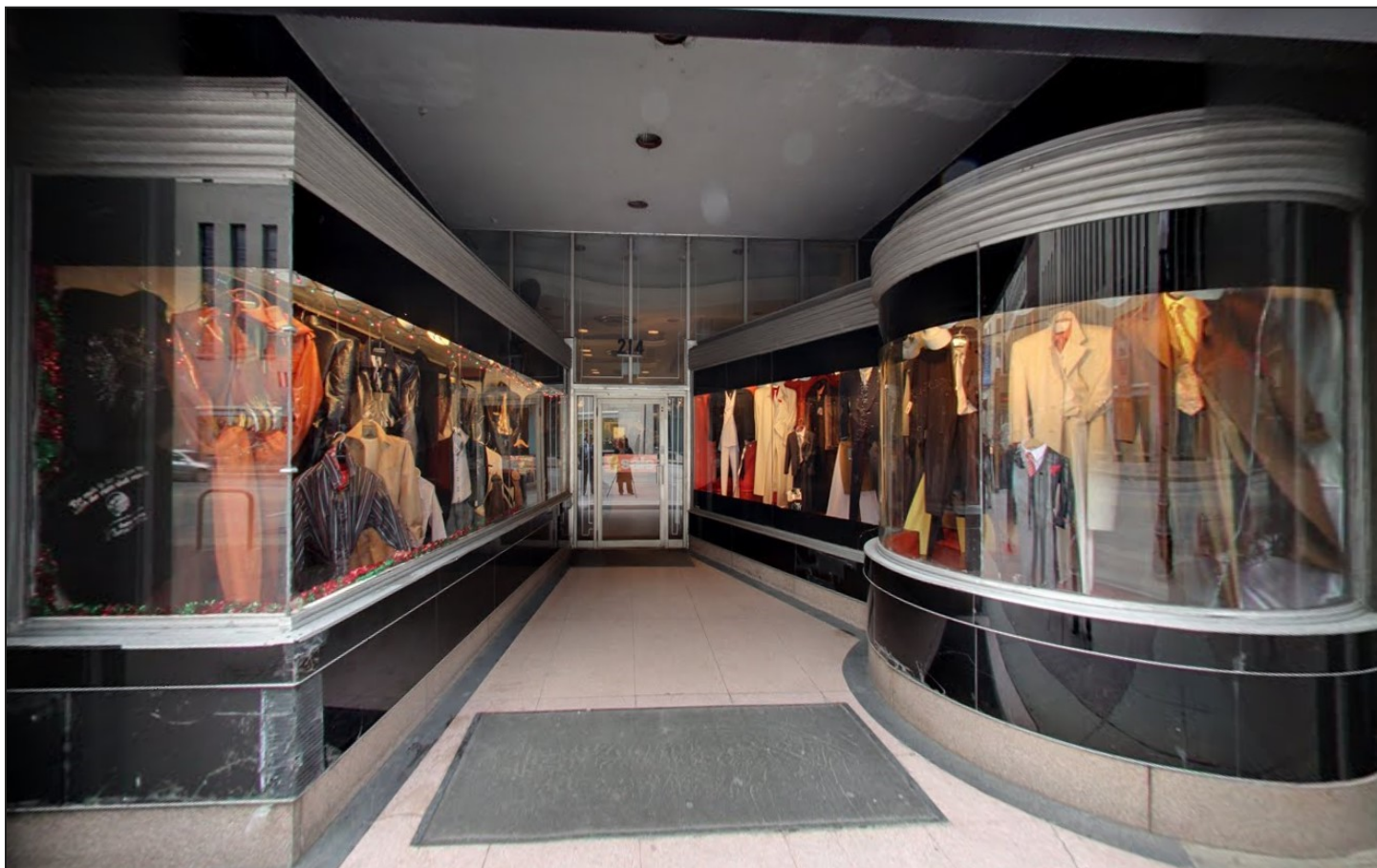
Roberto's storefront / originally Gunther's Confectionary, 214 S. State. Remodeled in 1949 by Isadore E. Alexander in a streamlined, high-style Art Moderne style. A highly intact and rare survivor celebrating State Street's rich history. Photo Credit: Google Maps
