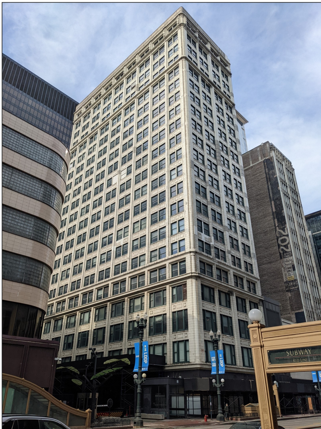
The Consumers Building, 220 S. State Street. Photo credit: Ward Miller / Preservation Chicago
