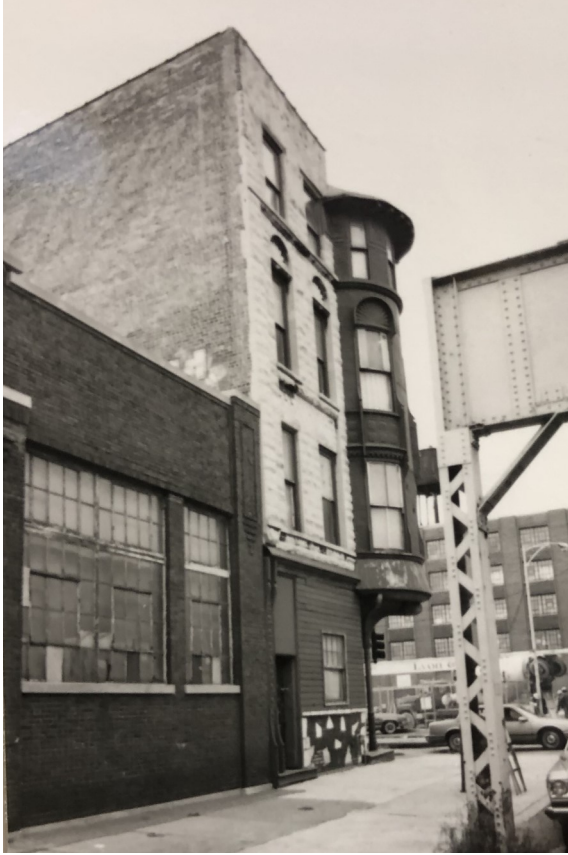
The north (Lake Street) and east (side) elevations of the (Former) Schlitz Brewery-Tied House located at 1393-1399 West Lake Street, 1987. The faded paint of a sign including the trademark Schlitz font logo can be seen on the east elevation. (Survey card, Chicago Historic Resource Survey )
