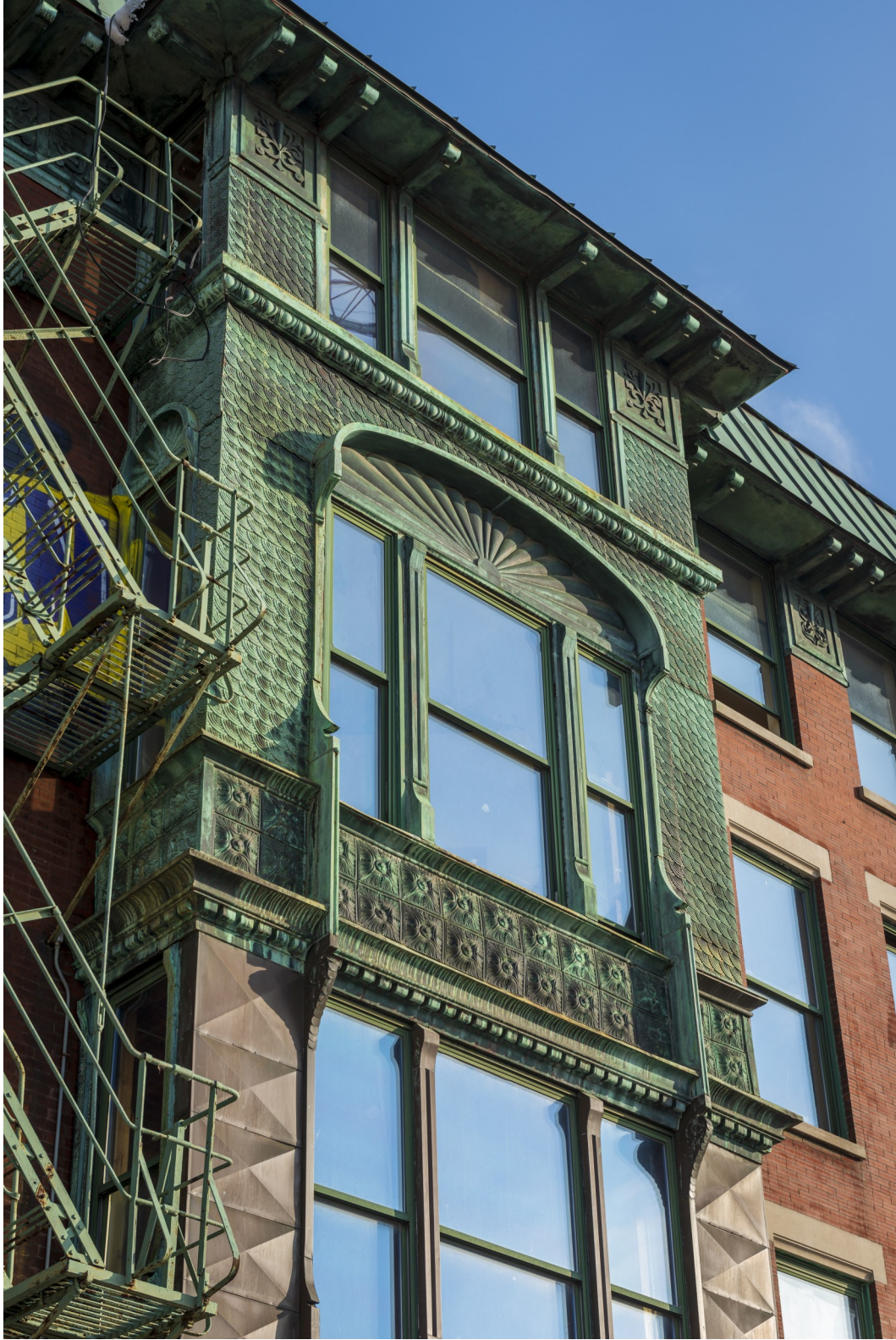
The bay window at the west elevation of the (Former) Schlitz Brewery-Tied House, 1393-1399 West Lake Street. Copper cladding features scalloped detailing with flower panels and a segmental arch lunette with decorative fan detail. Panels with an anchor-like detail trim the top of the bay window and continue along the entire elevation and turret just under the eaves. (Photo by Patrick L. Pyszka)
