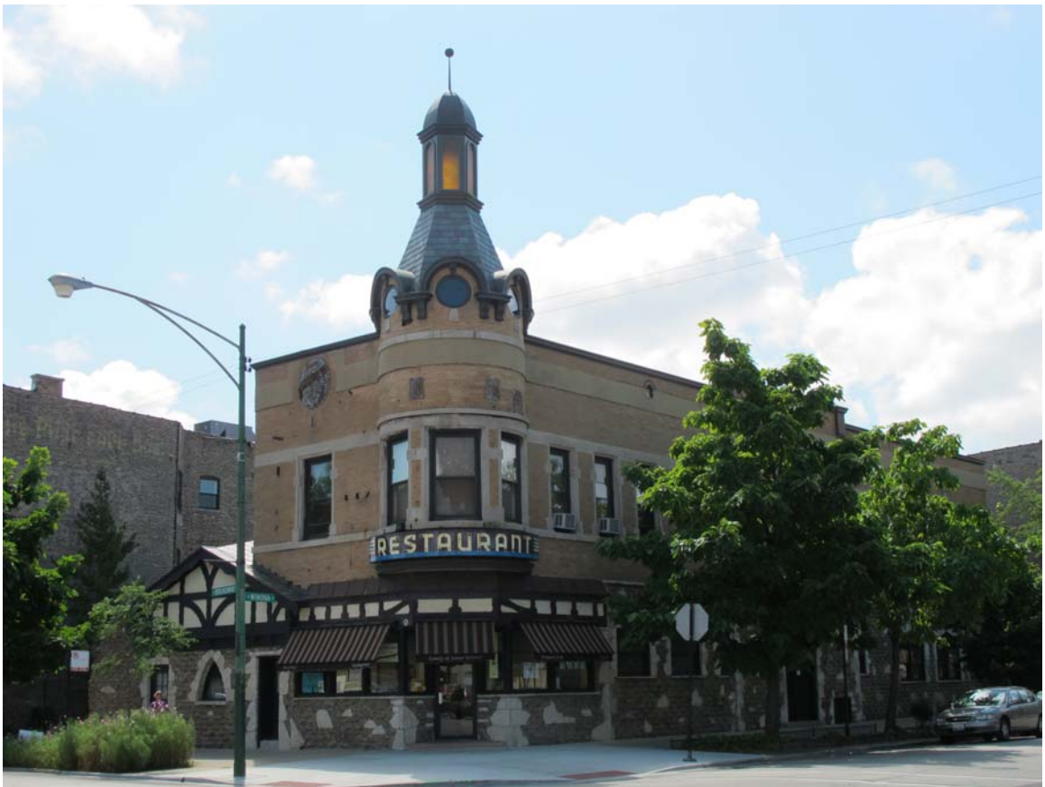
The Schlitz brewery-tied house at 5120 N. Broadway possesses excellent integrity. View of the building circa 1956 (top) and today (bottom).
