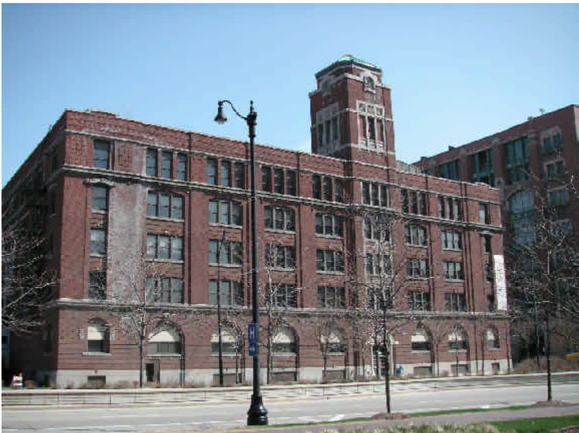
The nearly three-story masonry tower of brick, concrete, limestone and terra cotta concealed the building's water tanks and service tanks while providing a striking visual feature.
