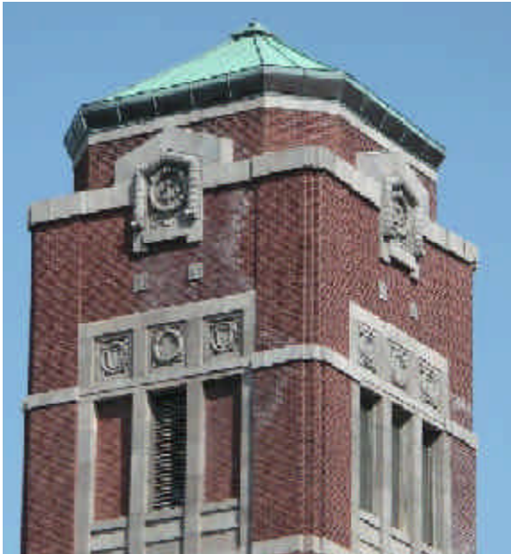
The nearly three-story masonry tower of brick, concrete, limestone and terra cotta concealed the building's water tanks and service tanks while providing a striking visual feature.
