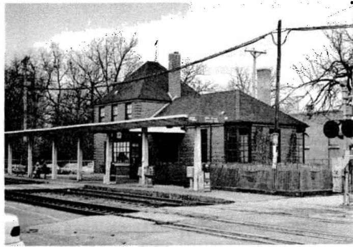
The youngest of the six stations, the 95th Street Station was built in 1945. The canopy was added in 1965.
