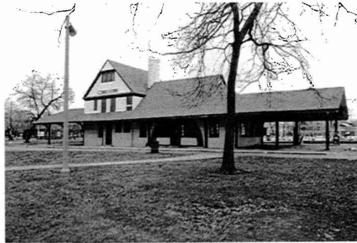
Fronting Bohn Park, the 111th Street Station is one of the most prominent features of the Morgan Park community.
