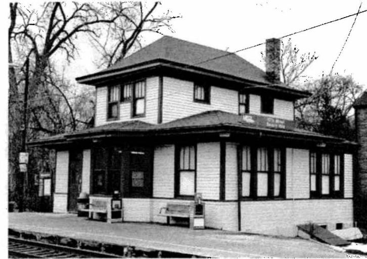
The design of the 107th Street Station (above) is similar to the scale of surrounding buildings, including nearby commercial structures (right).
