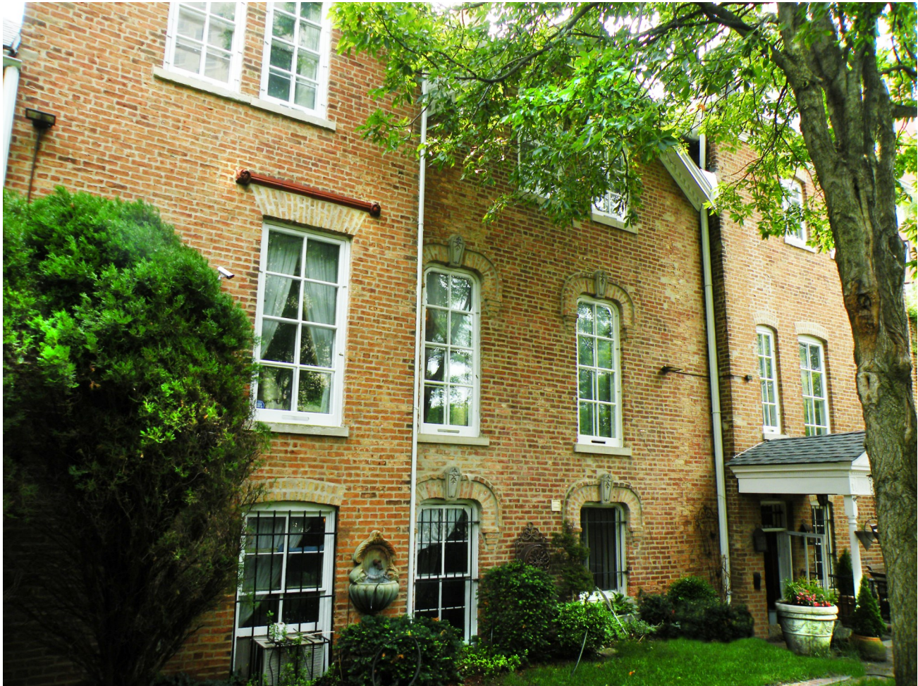
The west elevation of the Netterström House shows the west gable of the original house in the middle, between the 1890s corner tower addition on the left and the south addition on the right.
