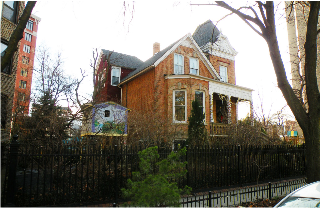
Above: The east and north elevations of the house. The frame east bay (red siding) is visible to the left.
