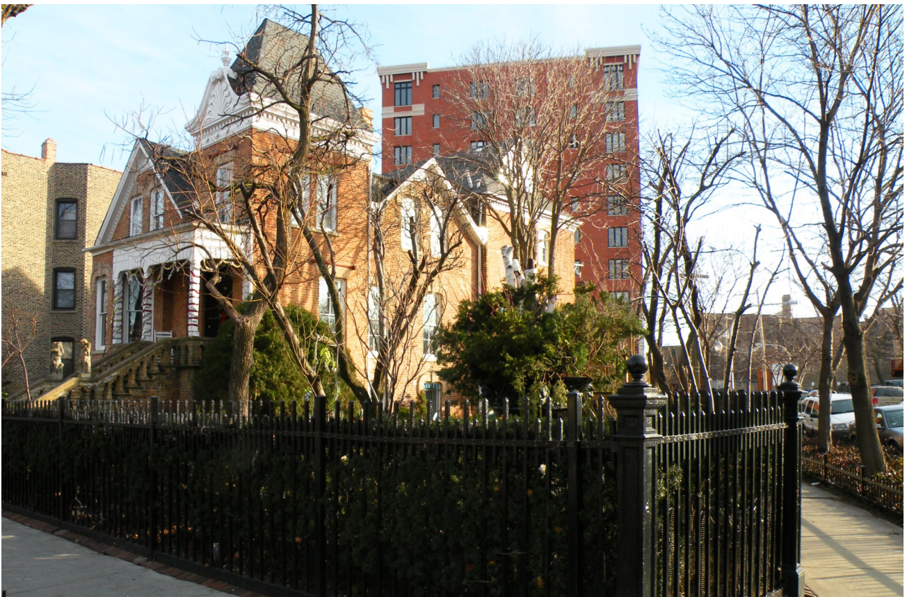
Below: The north and west elevations as viewed from the corner of Aldine Ave. and Dayton St.
