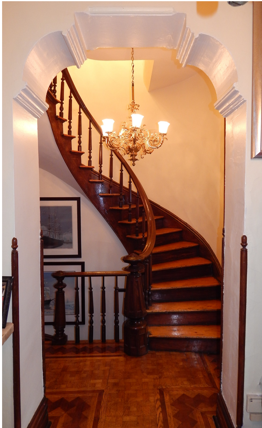
The main curving walnut and pine stair is part of the original portion of the house. In the foreground, the plaster archway leads from the may entry hall , which was built as part of the corner tower c. 1891-1894. The archway occupies the location of the original front door from before the corner tower was built.
