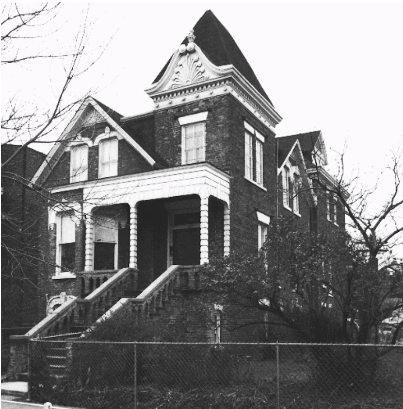
The Charles M. Netterström House was photographed at left in the 1980s for the Chicago Historic Resources Survey (CHRS). The house was given the second-highest color rating for architectural significance. At the time, the house's third owners, the Anderson family, lived in the house. They were also the house's longest occupants, owning the house from 1945 to 1994.
