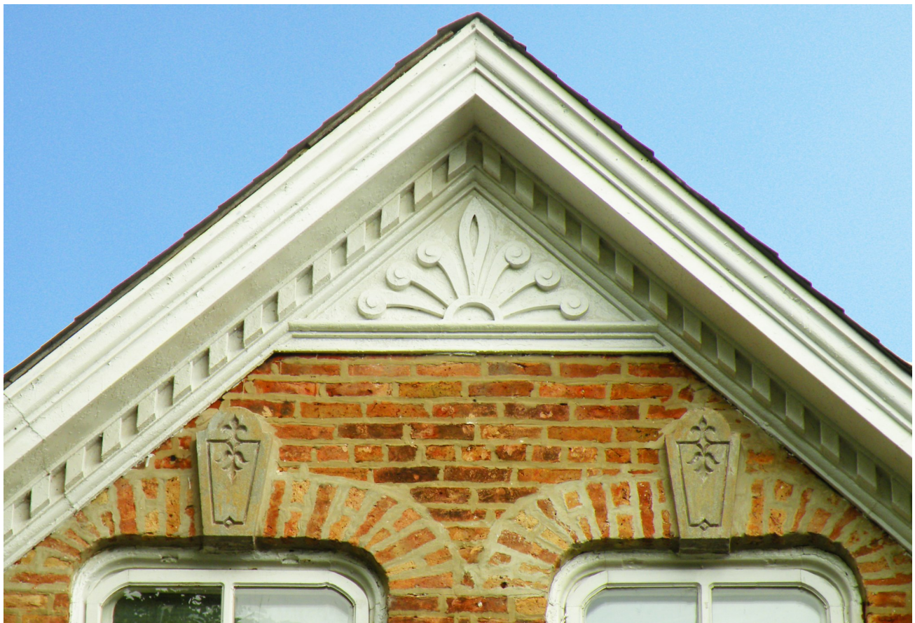
The north gable of the original portion of the house features cast stone keystones and a later Queen Anne style pressed metal cornice.
