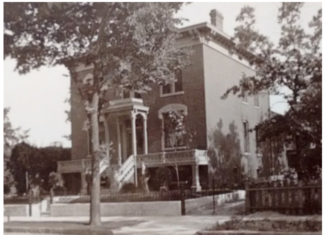
The Italianate-style home of Frederick Wesemann, built circa 1885 at what would today be 515 W. Briar Pl. Although Mr. Wesemann died in 1900, his widow is believed to have remained in the house until 1921. Chicago History Museum
