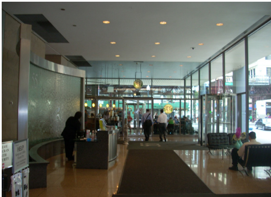
The Continental Center's original U-shaped lobby, which wrapped around three sides of the elevator core and featured unobstructed space, has been truncated by clear glass partition walls along its east and west ends. These partition walls separate the extant central lobby space from commercial and retail spaces on either side.
