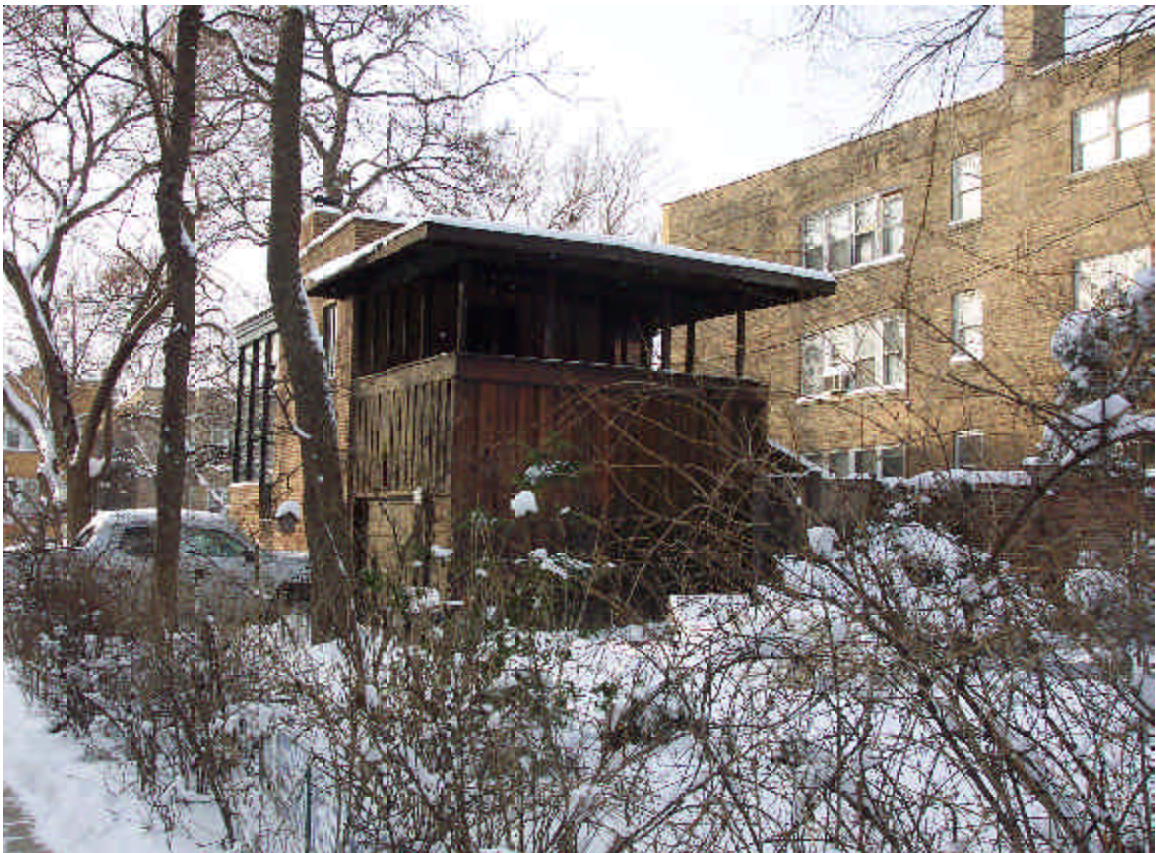
A view of the rear wood-sided garage and open-air roof deck of the Weintraub House.
