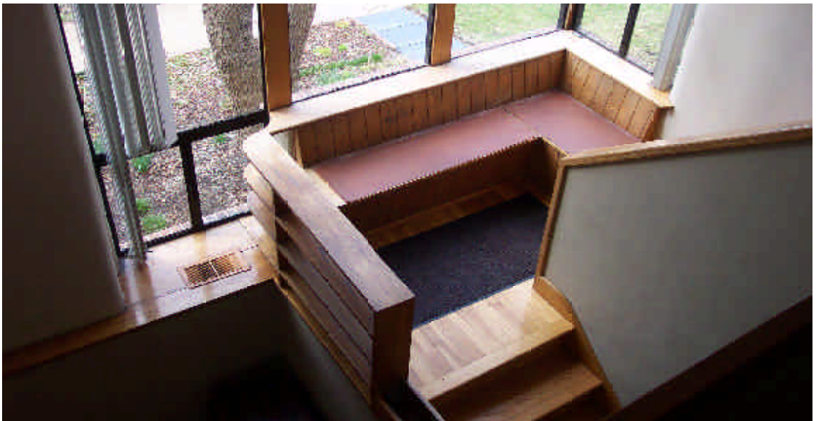
Two views of the stairwell from the second-floor corridor: (top) looking out towards the intersection of Victoria and Spaulding; and (bottom) down onto the window seat.
