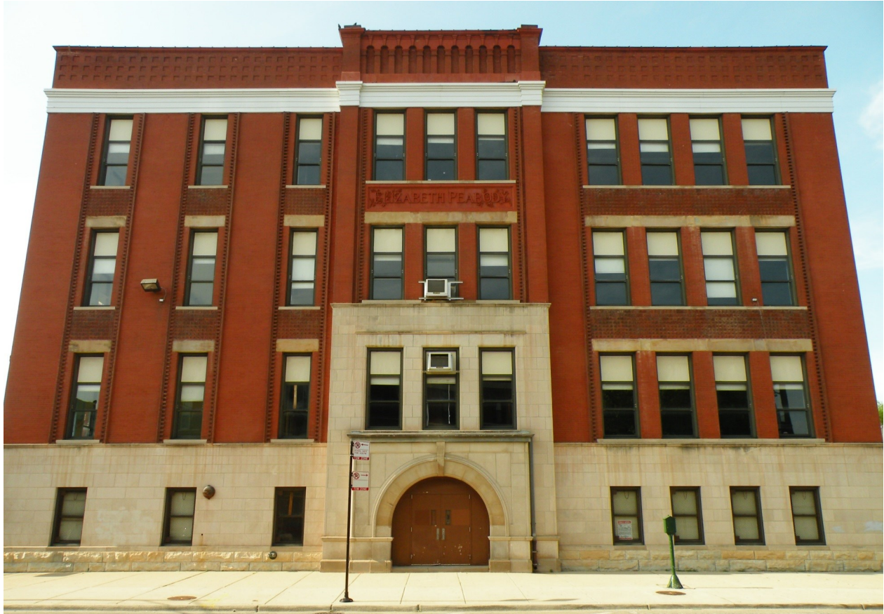
W. August Fiedler's 1894 Peabody school was one of his first designs. While maintaining the traditional tripartite design of base, middle, and crown, it blends older school building forms and styles with hints of modern new American Architectural styles.
