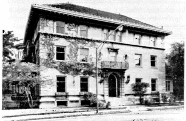
C. S. Roberts, who was in the coal business, was the first owner of this house at 4900 Ellis Avenue. The architects were Horatio Wilson and Benjamin Marshall who designed many residences in Kenwood. (Barbara Crane, photographer)
