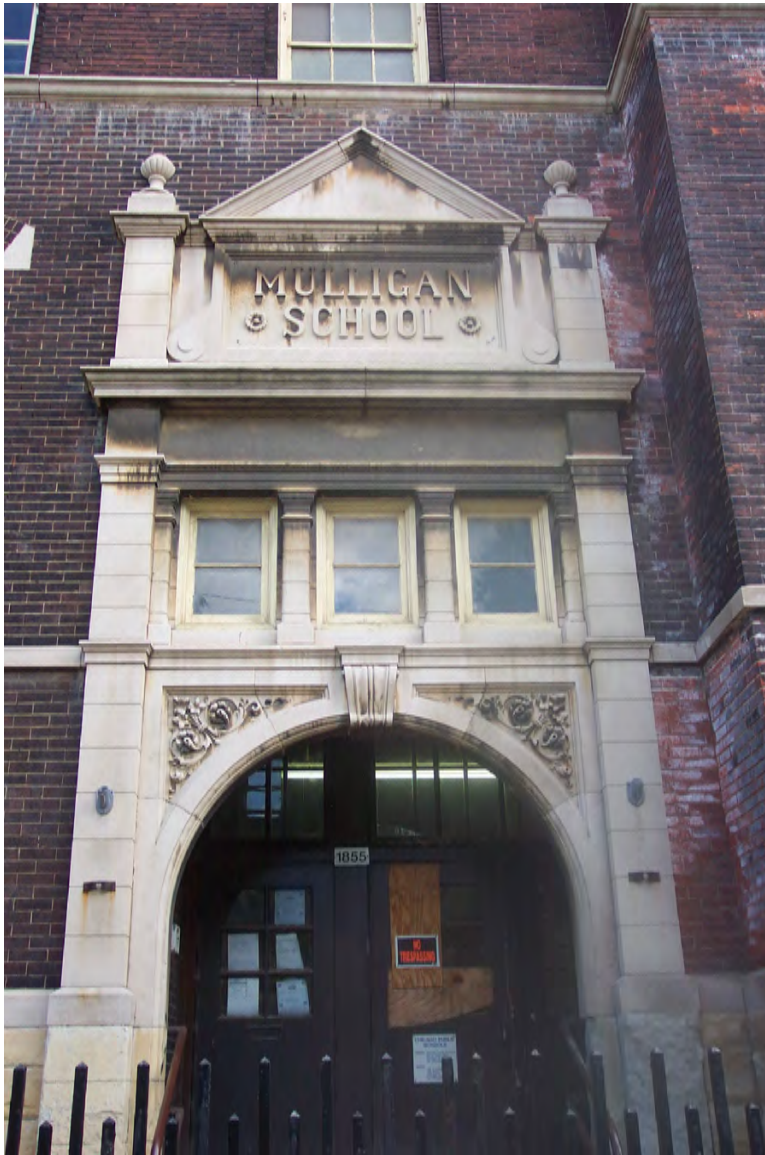
The entrance to the (Former) James Mulligan Public School Building is finely built of gray limestone and detailed with Classical-style ornament.
