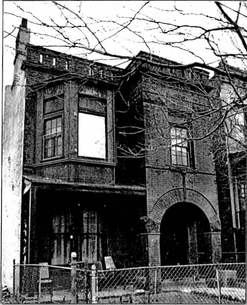
Figure 10: Residence, 4335 South Berkeley Avenue, built circa 1890. This design is particularly peculiar, having no basement, a ground-level porch, and a portal that is entered through the base of a second-story masonry bay. (Photograph by Timothy N. Wittman)
