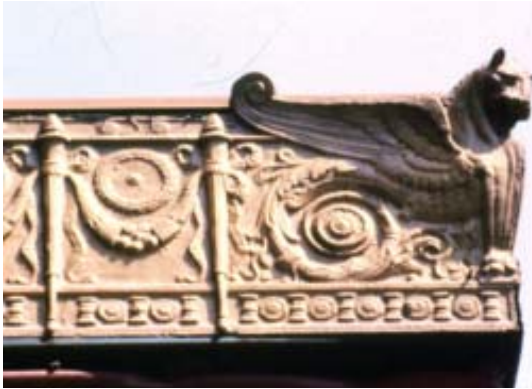
Left and middle: The entrance canopies of the Palmer House Hotel have bronze Classical-style ornament.
