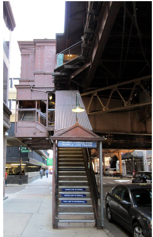
The west elevation of the west stationhouse (above) with the mezzanine level below it. The stationhouse exteriors are decorated with Neoclassical details (bottom left) rendered in pressed metal. Below right is one of the covered stairways which provide access to the Quincy Elevated Station.
