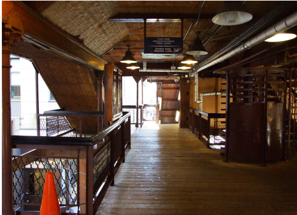
Top: The stationhouse interiors are embellished with pressed-metal wall and ceiling panels and varnished oak floors, wainscoting, and trim. Pictured is an interior view of west stationhouse at the Quincy Elevated Station.
