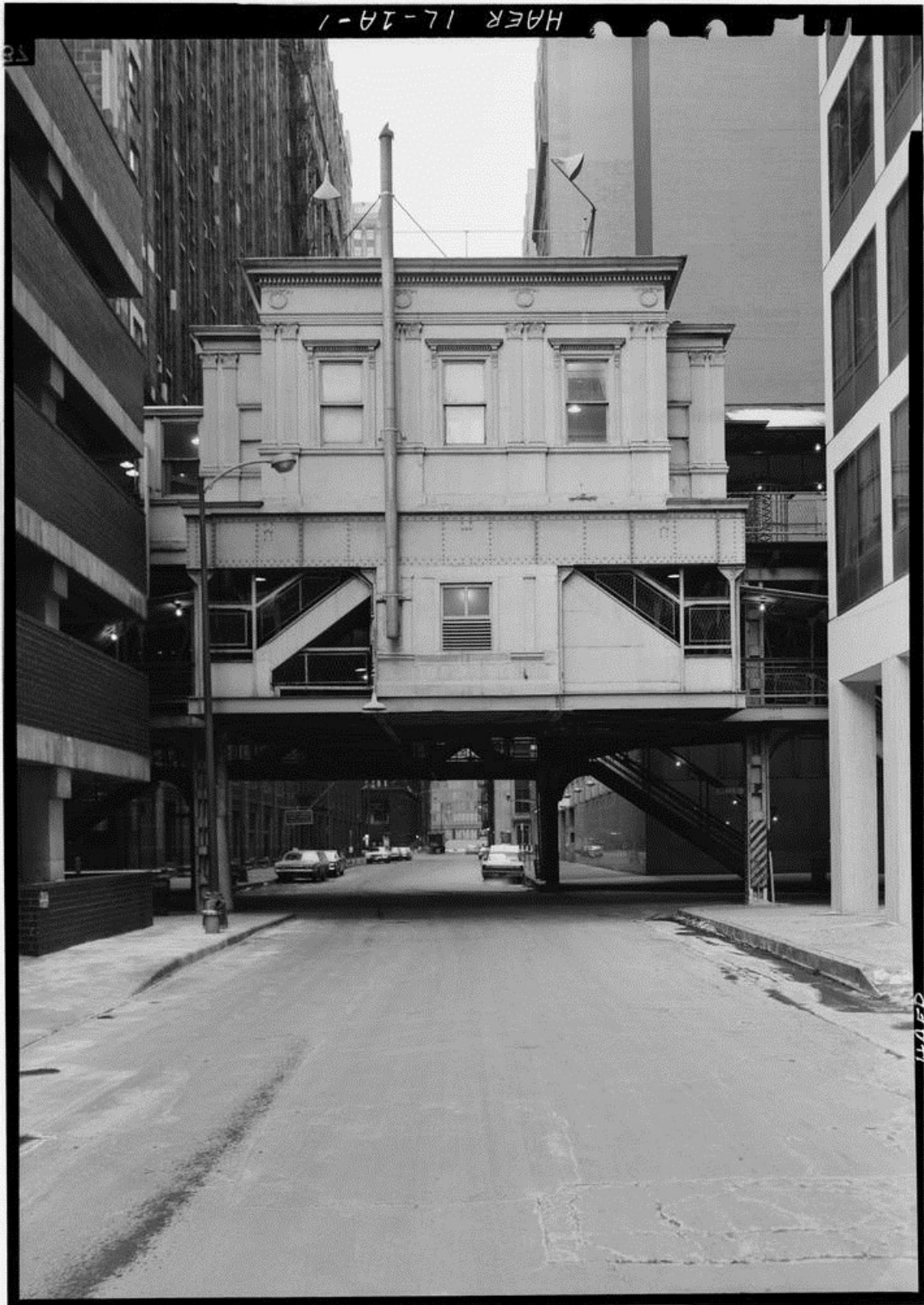
The Quincy Elevated Station in 1971, photographed by Jack Boucher, for the Historic American Engineering Record, Library of Congress.
