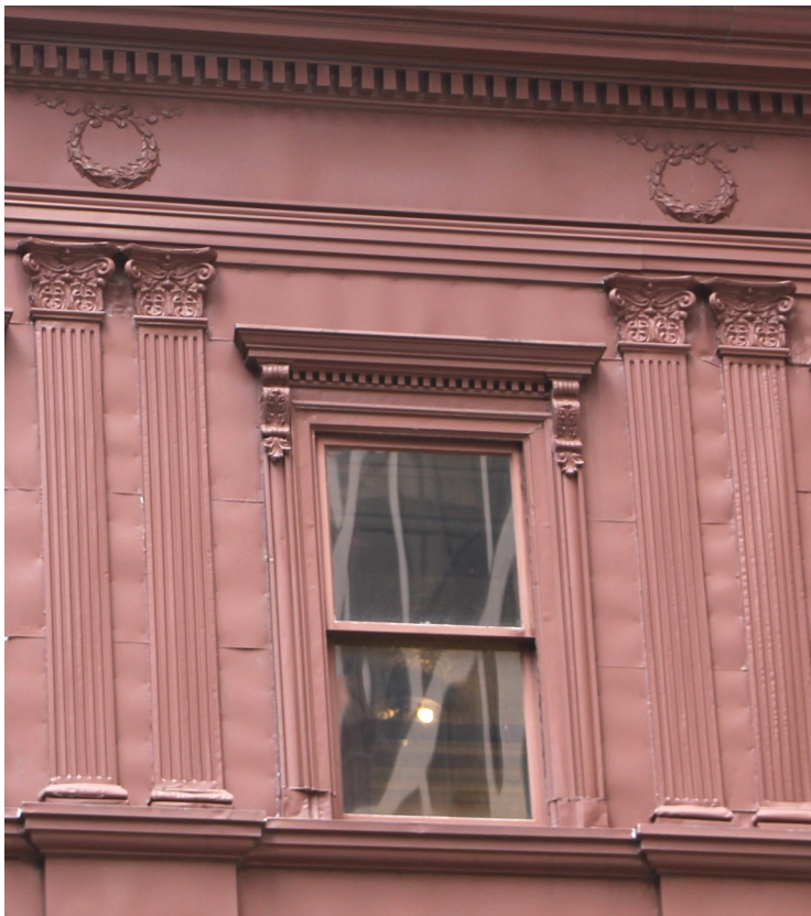
The west elevation of the west stationhouse (above) with the mezzanine level below it. The stationhouse exteriors are decorated with Neoclassical details (bottom left) rendered in pressed metal. Below right is one of the covered stairways which provide access to the Quincy Elevated Station.
