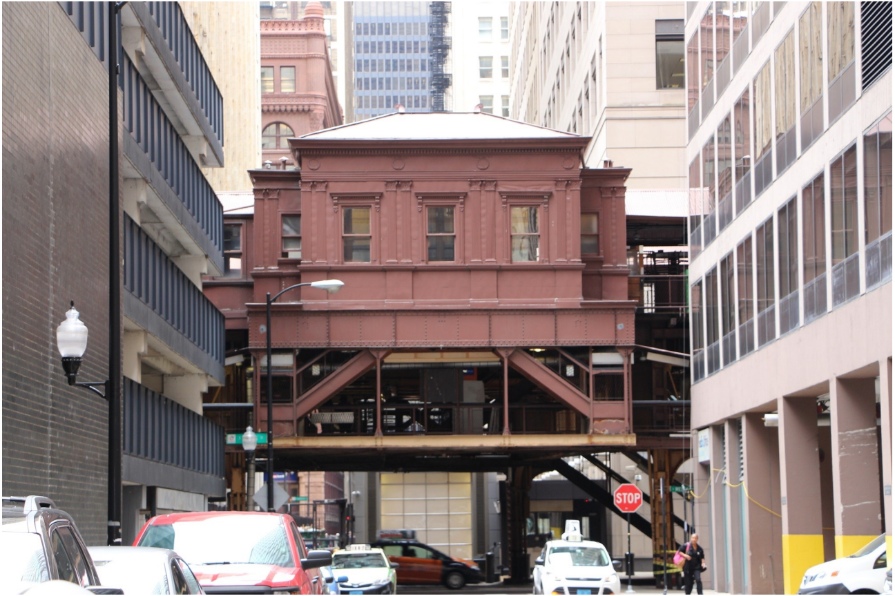
The west elevation of the west stationhouse (above) with the mezzanine level below it. The stationhouse exteriors are decorated with Neoclassical details (bottom left) rendered in pressed metal. Below right is one of the covered stairways which provide access to the Quincy Elevated Station.
