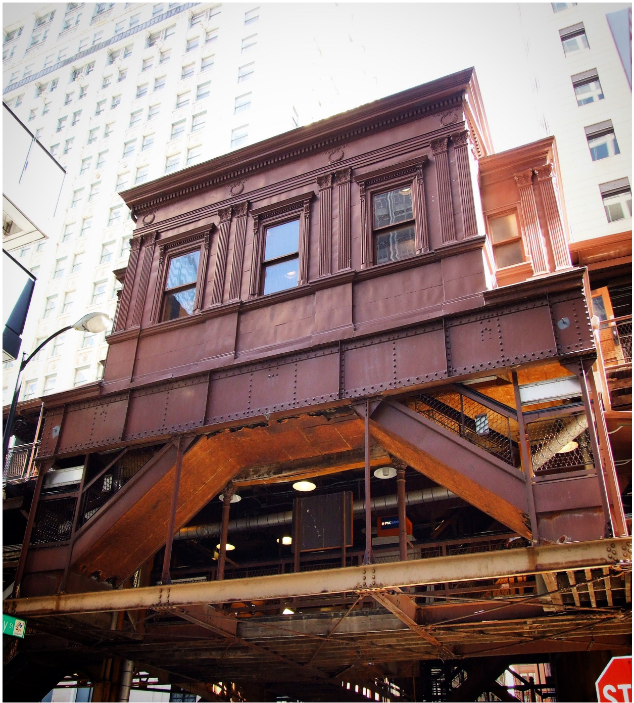
The street-facing elevation of the west stationhouse of the Quincy Elevated Station. The station is located at the intersection Quincy and Wells Streets in Chicago's Loop. The station was designed in the Neoclassical style with Palladian influences between 1896-1897. (McGuire Iglesias & Associates, Inc.)
