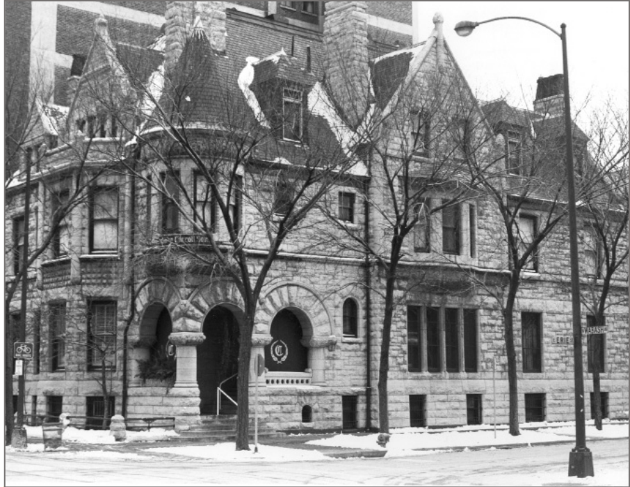
Still standing at 25 E. Erie, is the picturesque Richardsonian Romanesque style home also designed by Cobb & Frost in 1885. The recessed corner entry of this Chicago Landmark is distinguished by heavy round arches atop squat piers.
