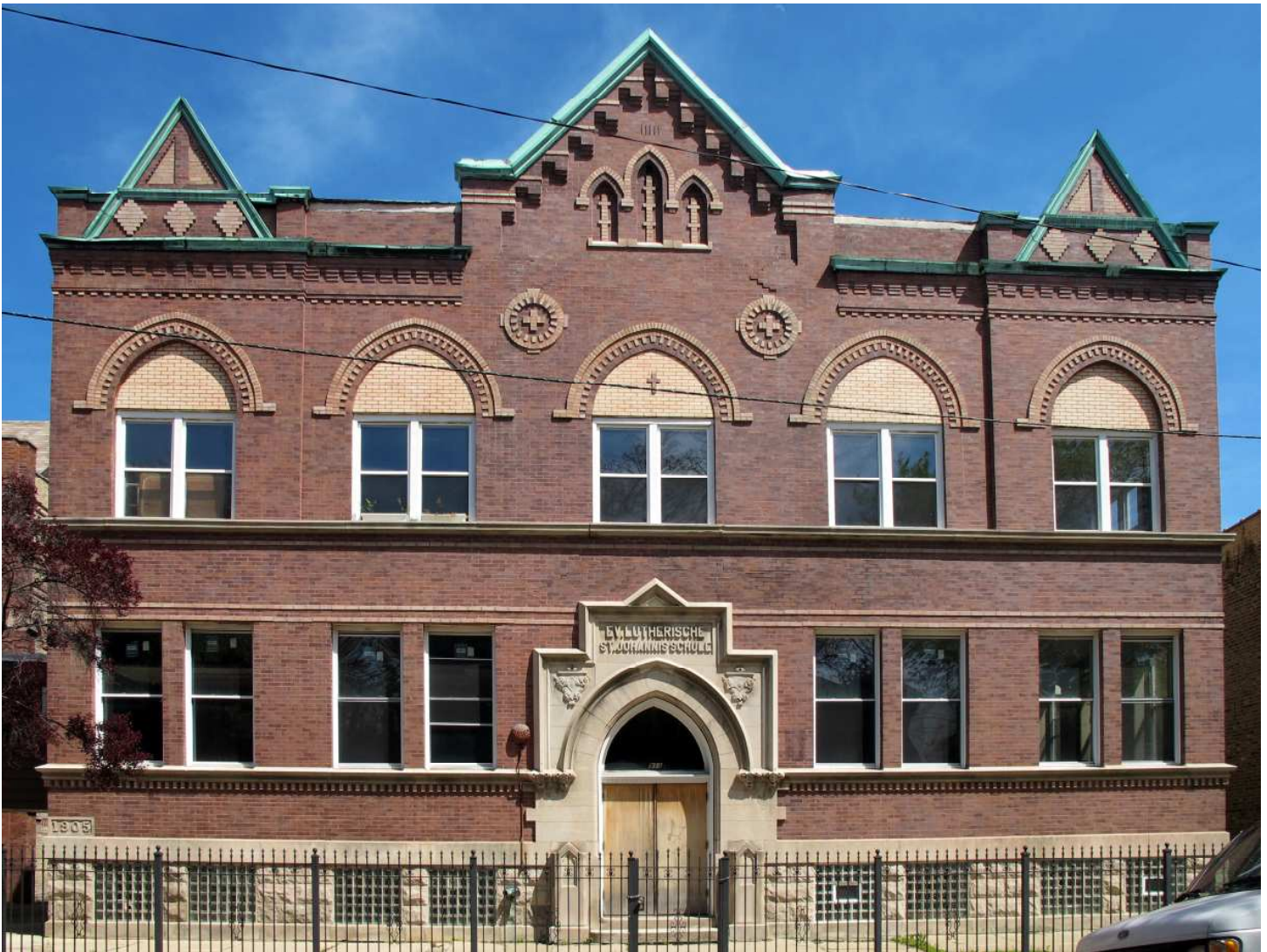
The St. John Evangelical Lutheran School Building employs fine brickwork and Gothic Revival motifs to form, with the Church Building, a visually unified parish complex.
