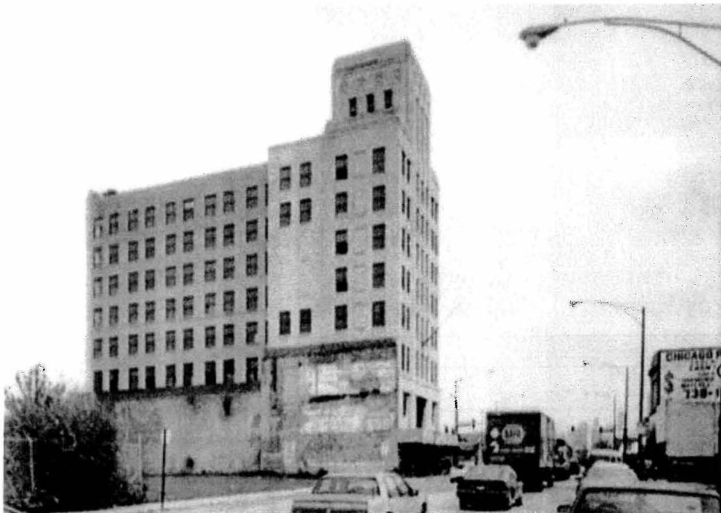
When completed in 1930, the West Town State Bank Building was part of the extensive commercial streetscape of West Madison Street, the West Side's most prominent shopping street. Top: A photograph from 1934 of W. Madison, looking east towards the bank building. Above: Today the building remains one of the few historic buildings along Madison.
