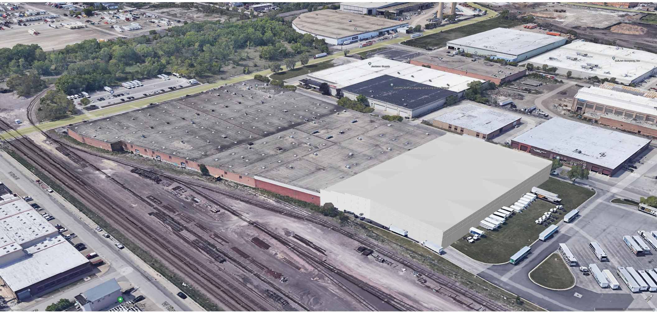
AERIAL VIEW OF SITE WITH MASSING OF THE EXPANSION: FROM SOUTH-EAST DIRECTION
