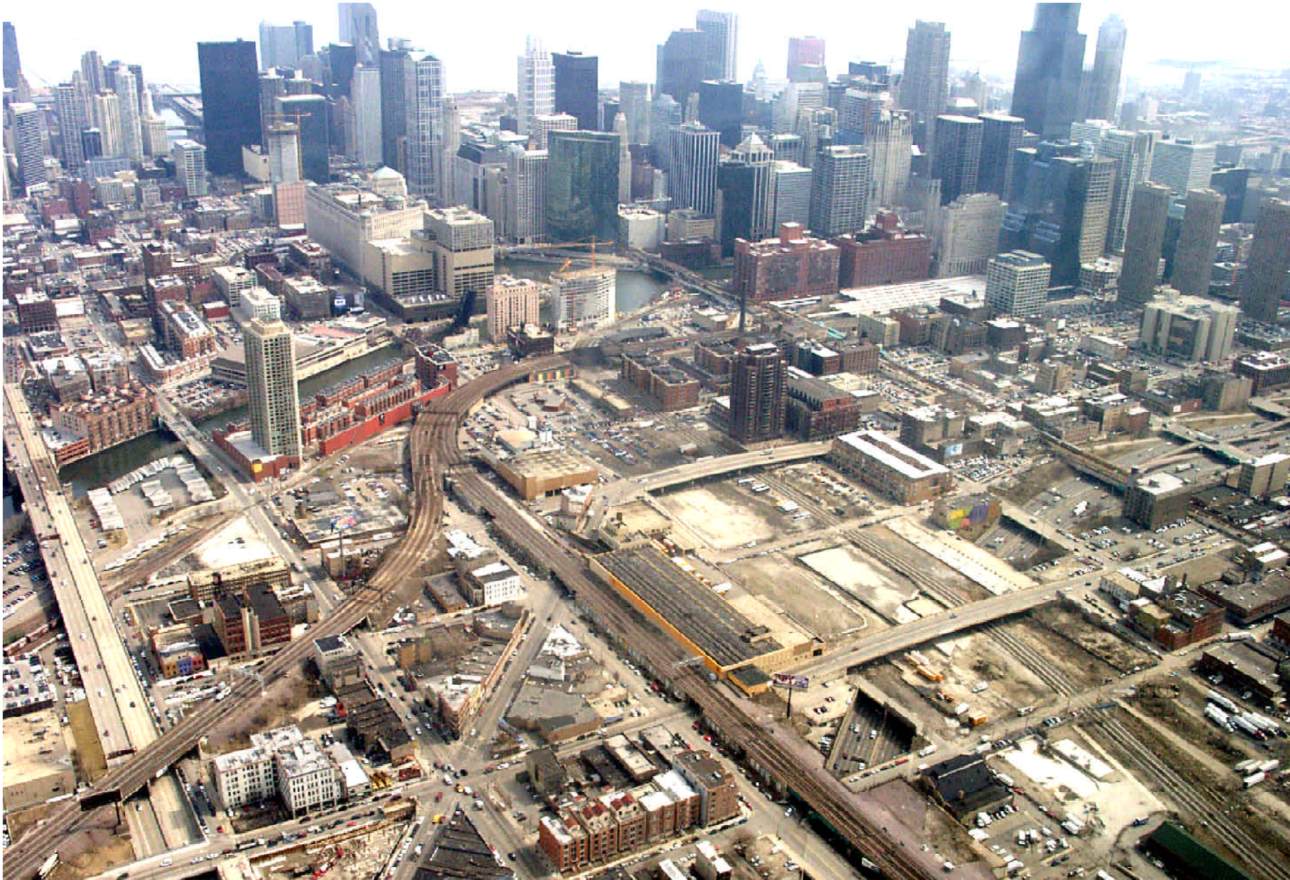
Figure 2.12 The Near Northwest offers potential for high density residential neighborhoods and enhancing existing industrial areas. Many of the rail easements offer potential for greenways extending from the Central Area to the West Side.
