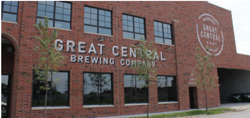
Example of new light industrial development orientation, massing, and scale. (221 N. Wood)
