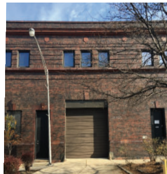
Loading and vehicle doors should also maintain the size of the original opening and consistency with other openings in the building.
