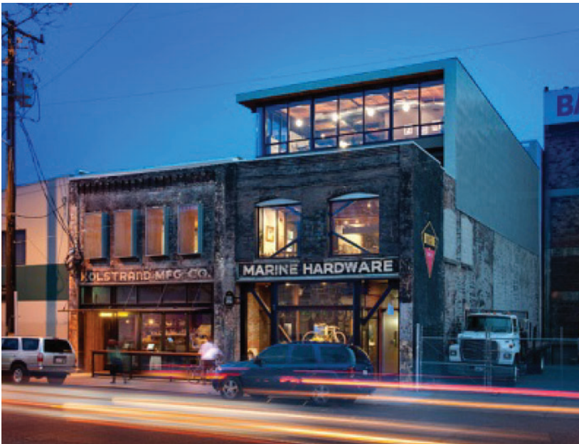
Example of an appropriate rooftop addition are set back from Ravenswood with floor heights compatible with existing building.
