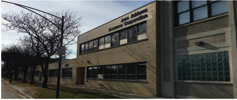
Continuous ribbon openings are common in buildings from the 1930s and 40s.
