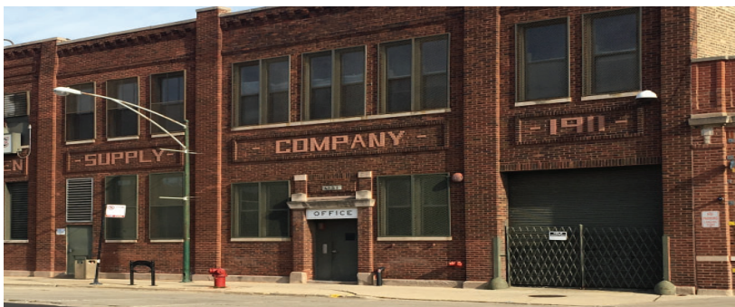
Original building signage should be retained where possible.
