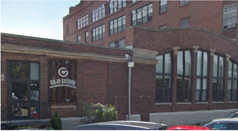
Example of an appropriate side and rear addition which incorporates durable materials found in the district including brick, limestone, and other materials compatible with the historic nature of Ravenswood Industrial Corridor.
