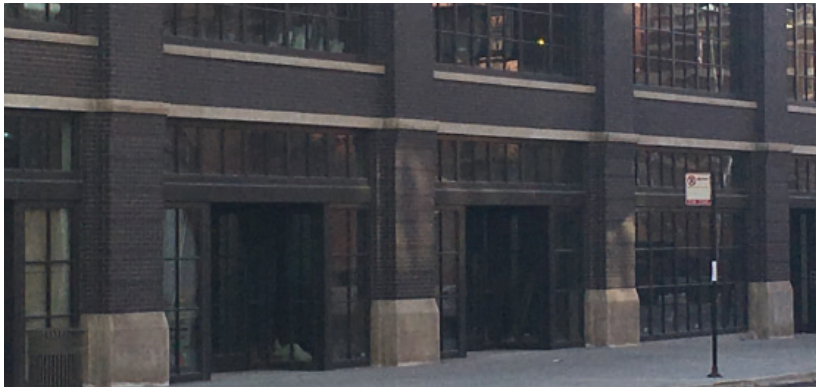
Example of new mixed-use office development incorporating brick, glass, and masonry materials (811 W. Fulton).
