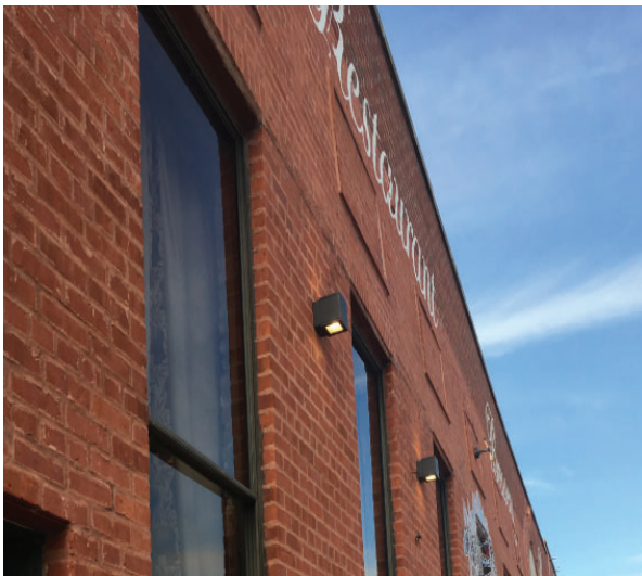
New exterior fixtures should be inconspicuous and appropriate to the industrial character of the Ravenswood Industrial Corridor.
