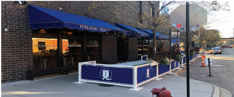
Canopies should be limited to the first floor and incorporate signage at the valance area only
