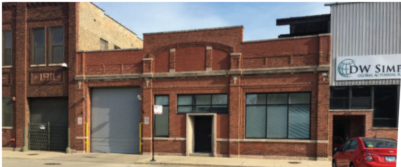
Decorative brick and stone features should be retained and restored.
