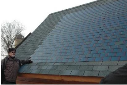
**Figure 10:** BIPV system, solar PV panels are built into the shingles of a roof (<a href="http://solarenergyfactsblog.com">http://solarenergyfactsblog.com</a>)
