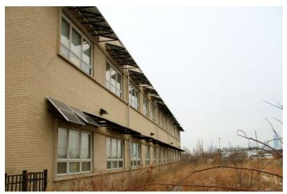
**Figure 7:** At the Chicago Center for Green Technology, solar panels serve a dual purpose, as they are used to generate electricity and are used as awnings above windows. This is an example of a non roof-mounted system. (Source: <a href="http://news.medill.northwestern.edu">http://news.medill.northwestern.edu</a>)
