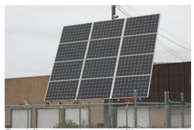
**Figure 9:** Single purpose pole-mounted solar PV system. (Source: <a href="http://www.mlive.com">http://www.mlive.com</a>)
