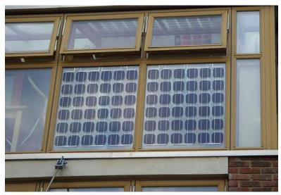
Figure 11: BIPV system, as a window of a structure (<a href="http://inhabitat.com">http://inhabitat.com</a>)
