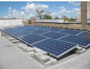
**Figure 5 (Above Left):** An example of a roof-mounted (penetrating) solar PV system (Source: <a href="http://www.solarserviceinc.com">http://www.solarserviceinc.com</a>)
