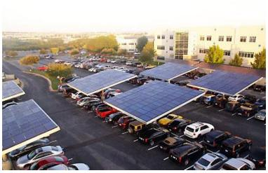
**Figure 8:** Dual purpose ground-mounted solar PV system located on a parking shading structure. (Source: <a href="http://climateinc.org">http://climateinc.org</a>)
