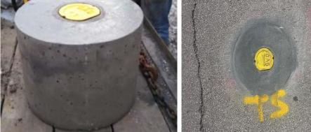
Keyhole technology is a method of accessing and viewing below grade utilities using small holes ("keyholes") using vacuum excavation in soft surfaces and traditional coring in hard surfaces. Typically, the keyholes are created for the purpose of subsurface utility investigation, pothole/depth checks or facility leak detection or repair; pavement restoration must follow specific guidelines set forth in this section.
