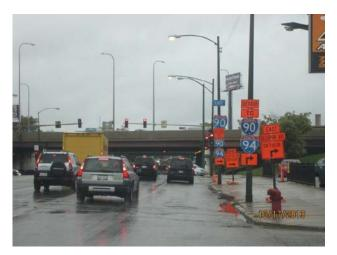
warning area. Spacing of the signage in the advance warning area is variable and determined by the speed limit. Refer to the table below for advance warning area sign spacing, unless otherwise approved by CDOT DOIM:
