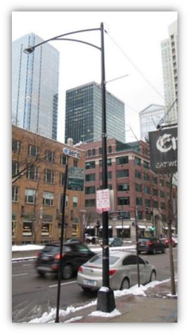
31' Ballast Housing Base Pole [This type of steel pole is being phased out, Replacement pole CDOT Spec 808]
