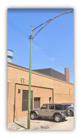
Legacy Streetcar System Span Pole [This type of steel pole is being phased out, Replacement pole: CDOT Spec 808]
