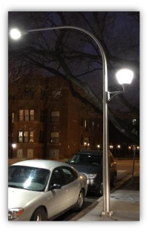
20 Ft. Steel Legacy Residential Light Pole [This type of steel pole is being phased out, Replacement pole: CDOT Spec 808]
