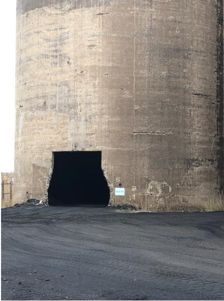
Figure 3 - IRM Process Silo
