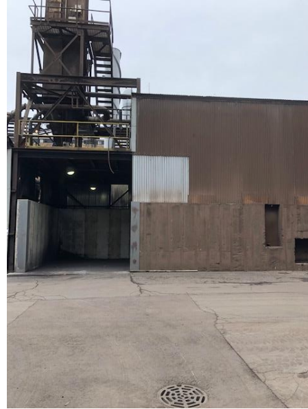
Figure 4 - "8-9 Junction" Building with Baghouse
