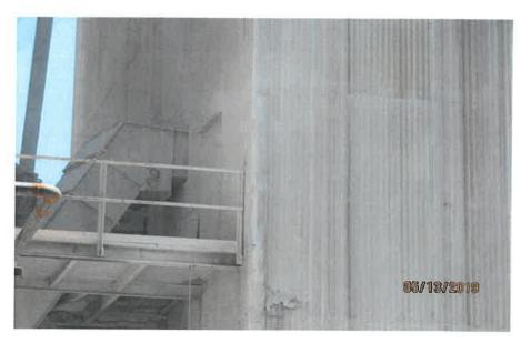
COMMENTS: Photo # 17Direction: SE Comments: Emissions of particulate dust from openings on wall, door, pipes of
