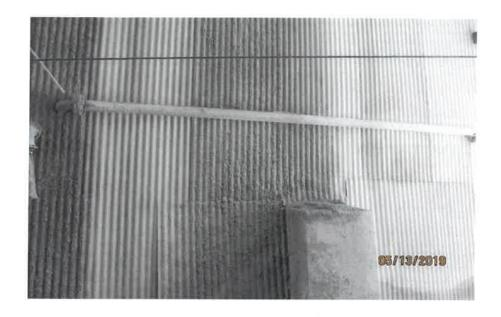
COMMENTS: Photo # 06 Direction: SW Comments: Accumulation of particulate dust on the ground, outside BC # 3 (rail car loading station building) & BC # 10. Also on walls, beams, pipes & other outside structures.
