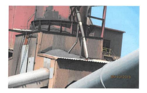
COMMENTS: Photo # 01 Direction: NW Comments: Accumulation of coke material on the roof of coke loading station.
