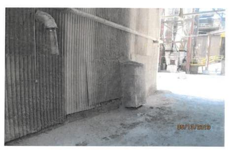
COMMENTS: Photo # 05 Direction: SW Comments: Accumulation of particulate dust on the ground, outside BC # 3 (rail car loading station building) & BC # 10. Also on walls, beams, pipes & other outside structures.
