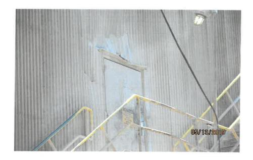
COMMENTS: Photo # 19 Direction: SE Comments: Emissions of particulate dust from openings on wall, door, pipes of BC # 3 (rail car loading station building) and BC # 10 building.
