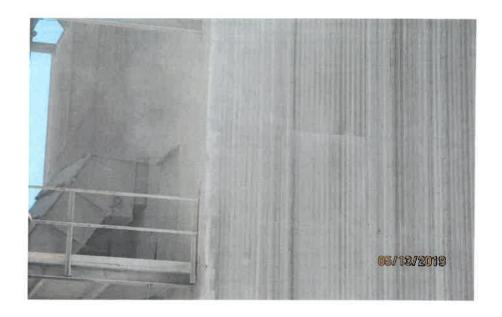
COMMENTS: Photo # 08 Direction: SE Comments: Emissions of particulate dust from openings on wall, door, pipes of BC # 3 (rail car loading station building) and BC # 10 building.
