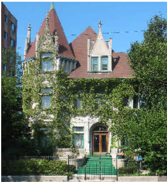
Griffiths-Burroughs House 3806 S. Michigan Avenue
