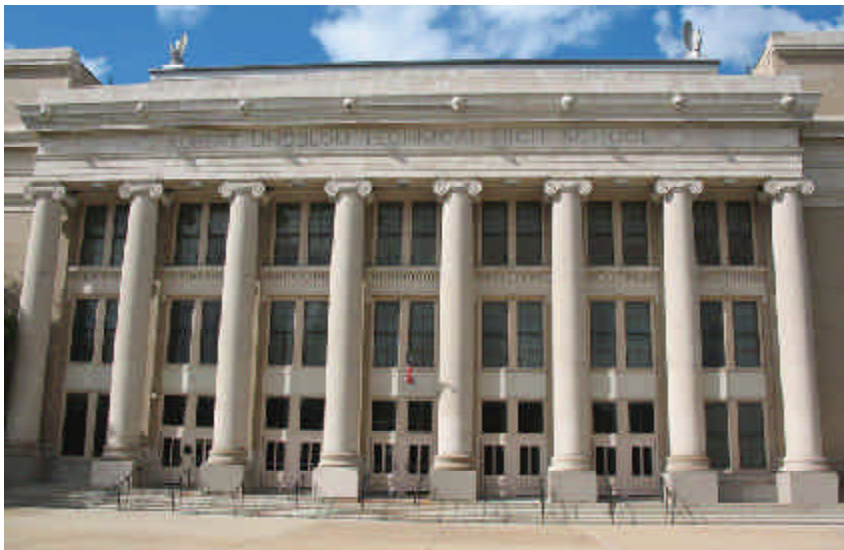
Lindblom Technical High School 6130 S. Wolcott Avenue
