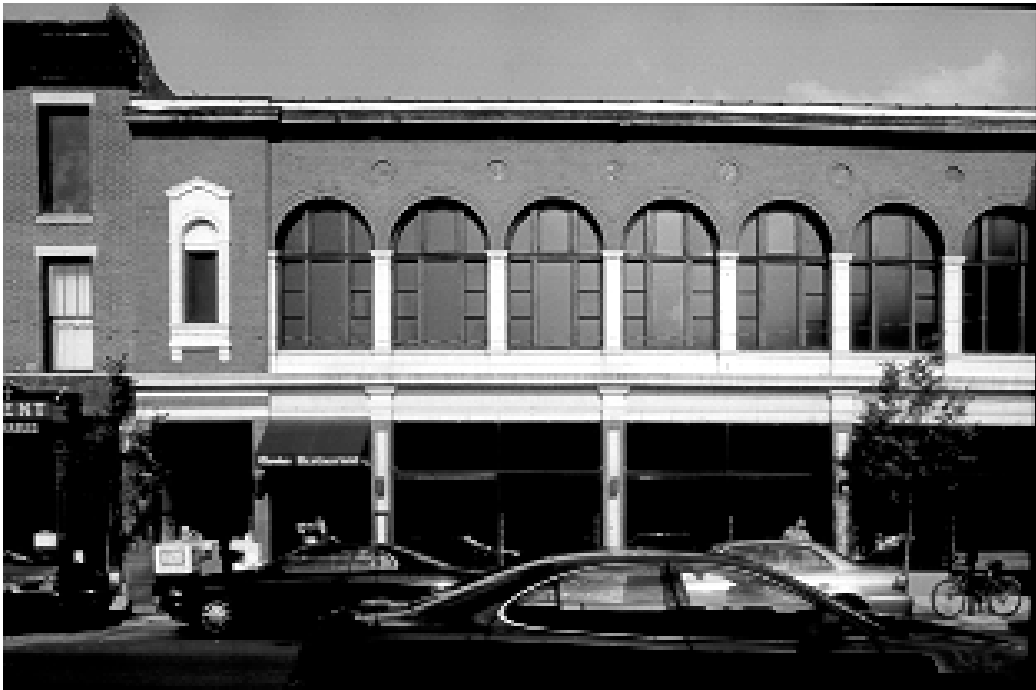
The Biograph Theater is one of the oldest theaters in Chicago expressly built to show movies. Its facade is handsomely detailed with a Palladian-style window (top, seen above the metal marquee) and a row of round-arched windows set within contrasting red brick and white terra cotta (above).
