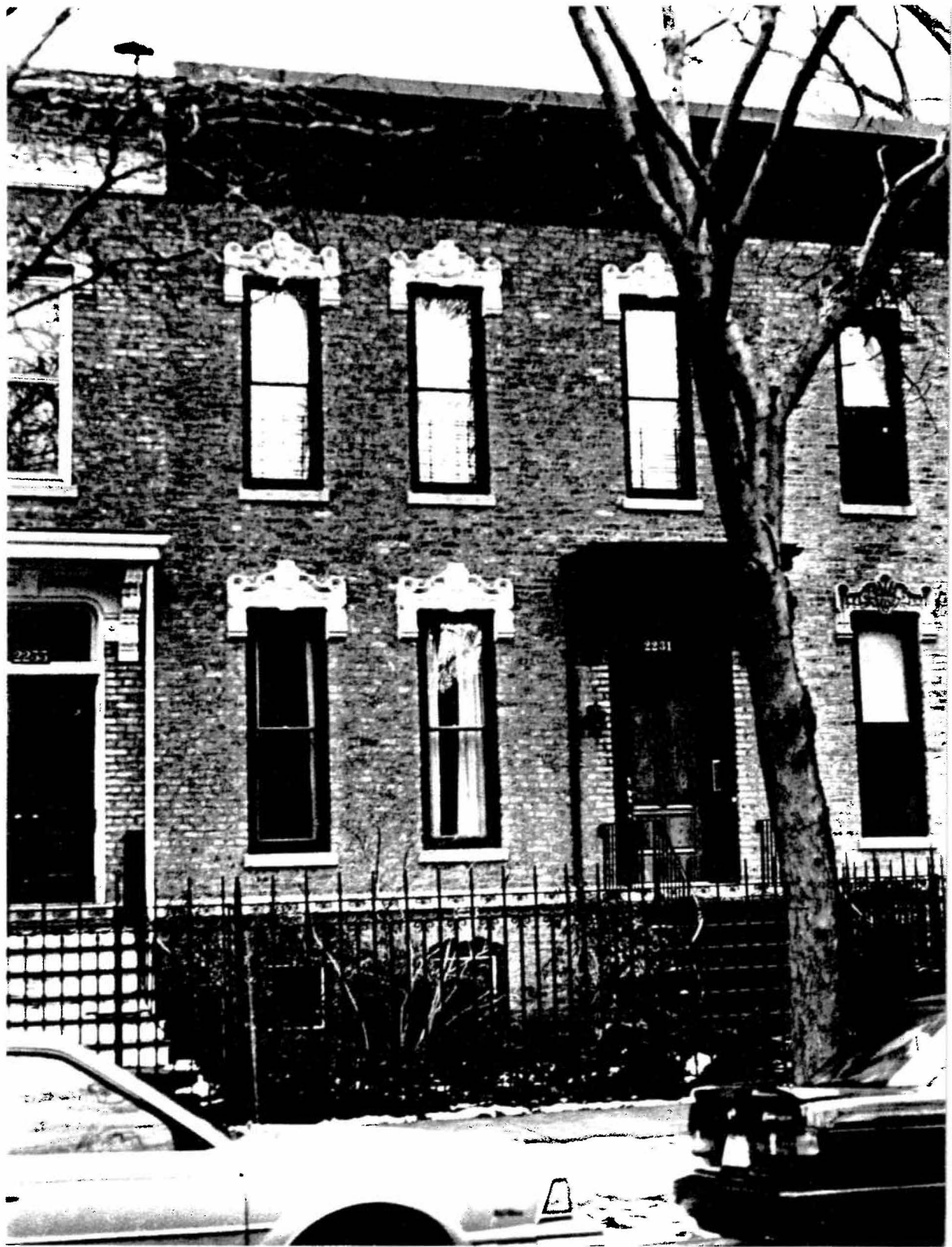
The row house at 2231 N. Burling St., shown above in a 1992 photograph, has the distinctive physical features of the houses in the Burling Row House District, including tall, narrow windows, stone lintels, and wood cornice.
