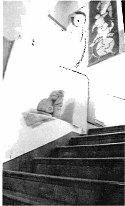
The Center's staircase, which was remodeled in 1940, is indicative of the New Bauhaus' design approach.
