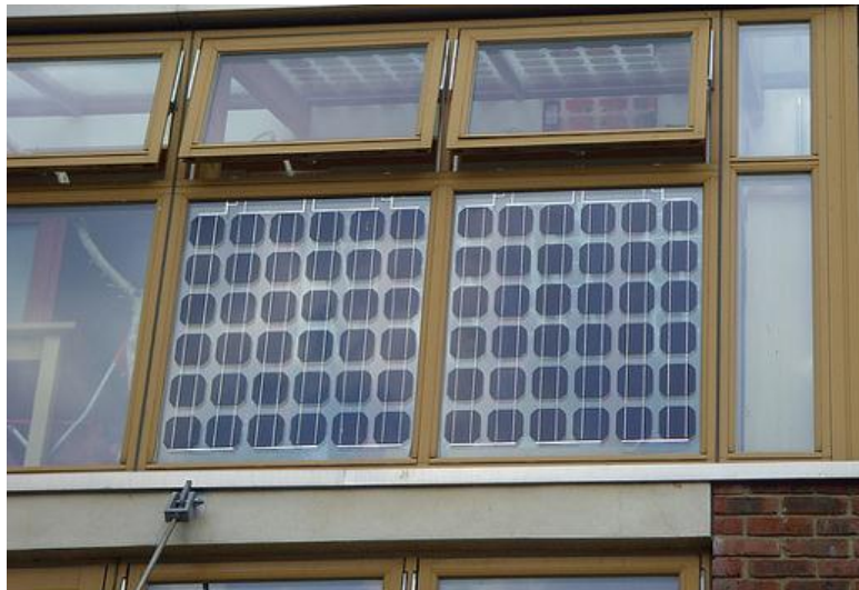
Figure 11: BIPV system, as a window of a structure ( http://inhabitat.com )
