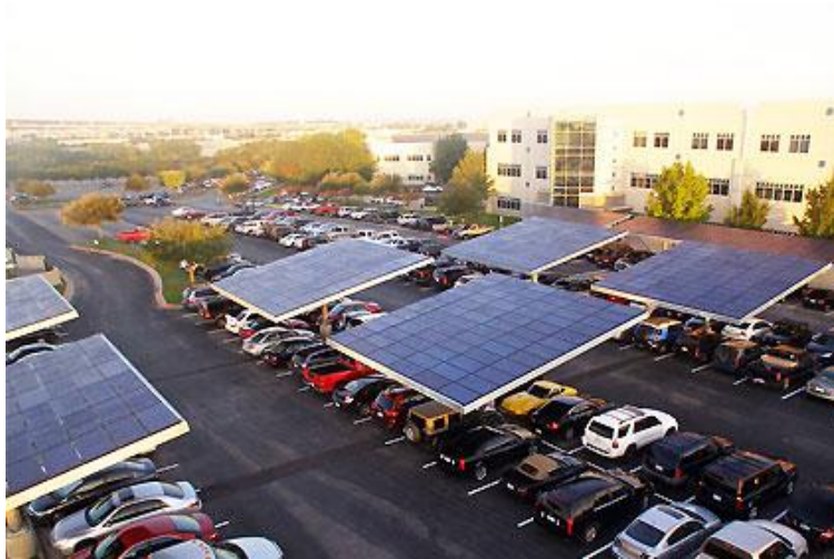
Figure 8: Dual purpose ground-mounted solar PV system located on a parking shading structure. (Source: http://climateinc.org )
