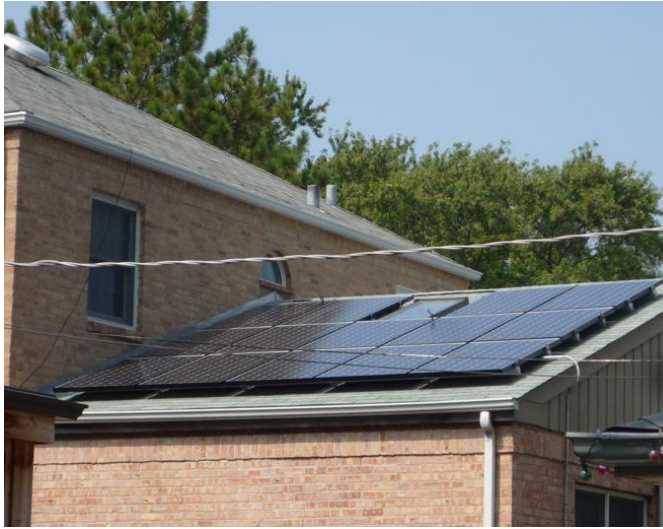
Figure 5 (Above Left): An example of a roof-mounted (penetrating) solar PV system (Source: http://www.solarserviceinc.com )
