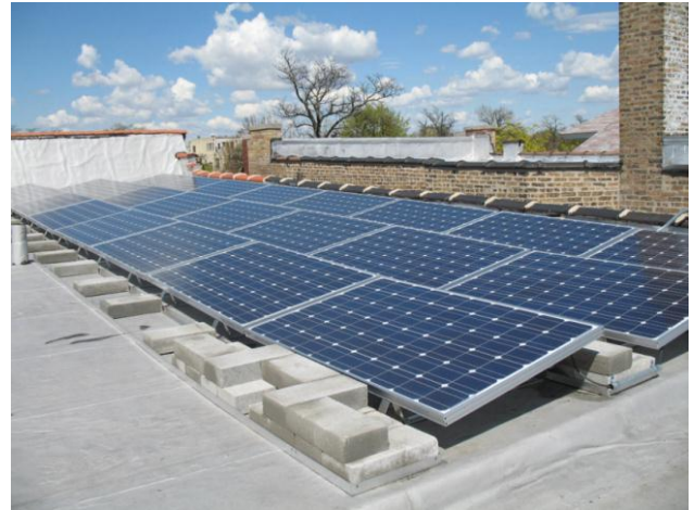
Figure 5 (Above Left): An example of a roof-mounted (penetrating) solar PV system (Source: http://www.solarserviceinc.com )
