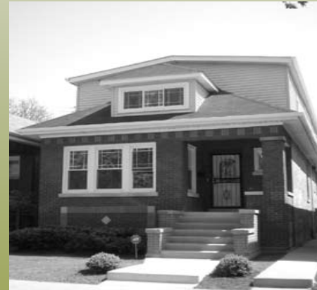
After NSP Rehab
