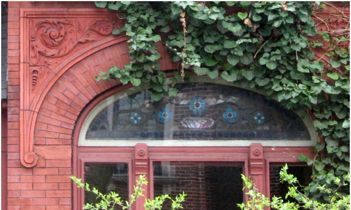
Details of terra-cotta ornament flanking the projecting bay's stained-glass transom.
