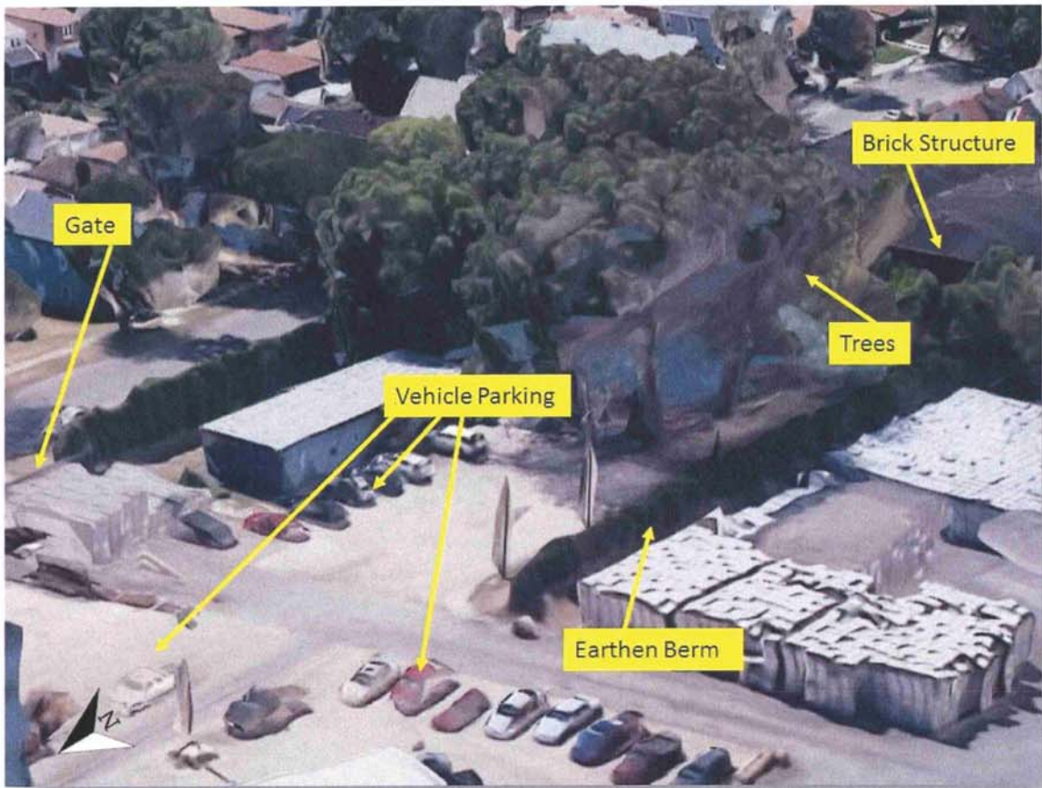
Figure 2 PS2.1 (Office Area) Site Layout S.H. Bell Facility, 10218 South Avenue O, Chicago, Illinois 60617
