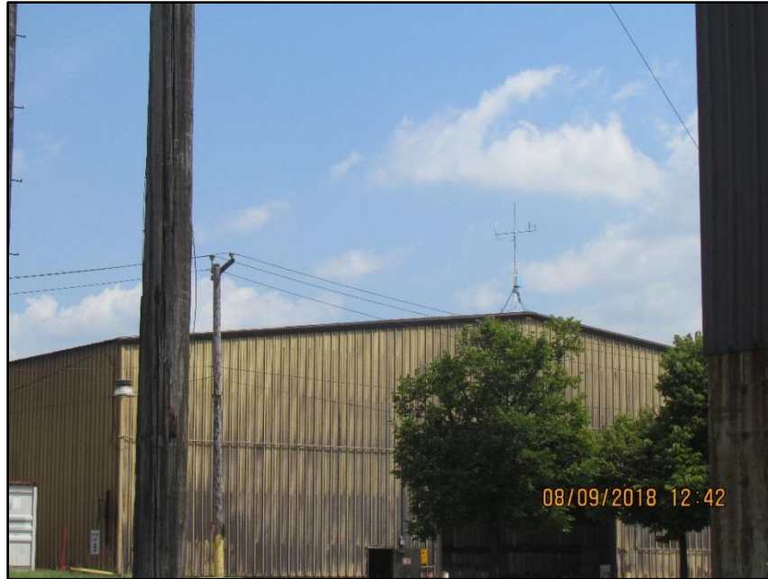
Figure 1.3 Photograph of Meteorological Tower on Building D
