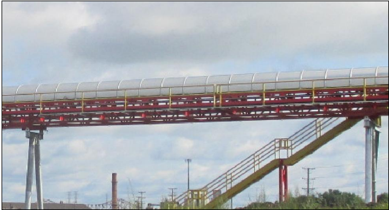
Figure 12 – Side View of a Typical Covered External Fixed Conveyor
