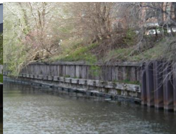
slopes on top of seawall
