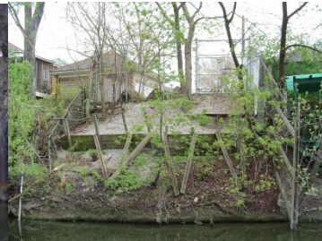
walls on top of slopes
