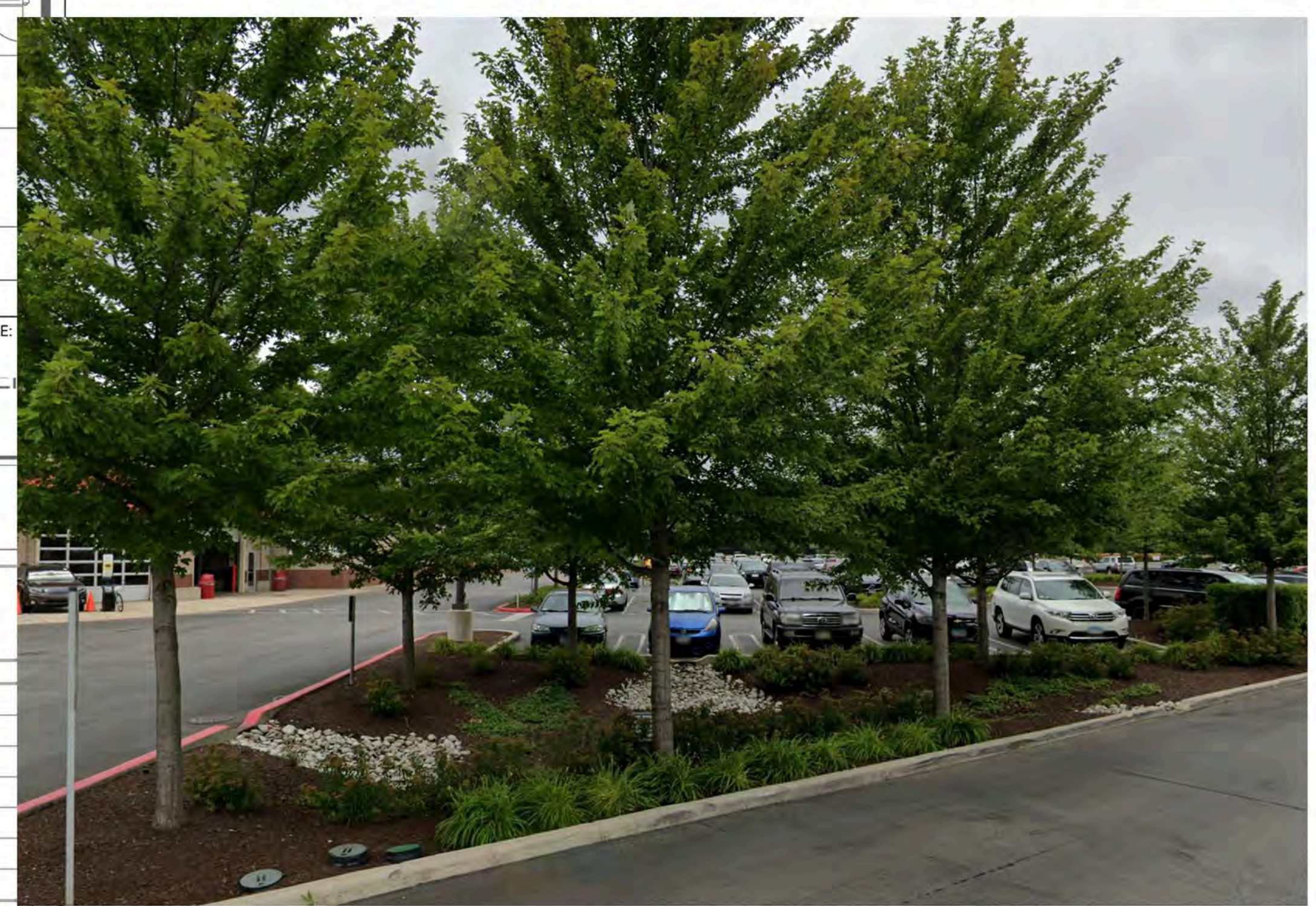
View at Existing Bioretention Basin
