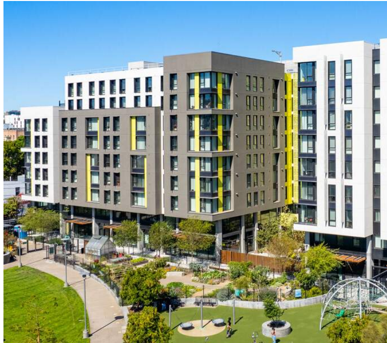
CASA ADELANTE AFFORDABLE HOUSING SAN FRANCISCO, CA
