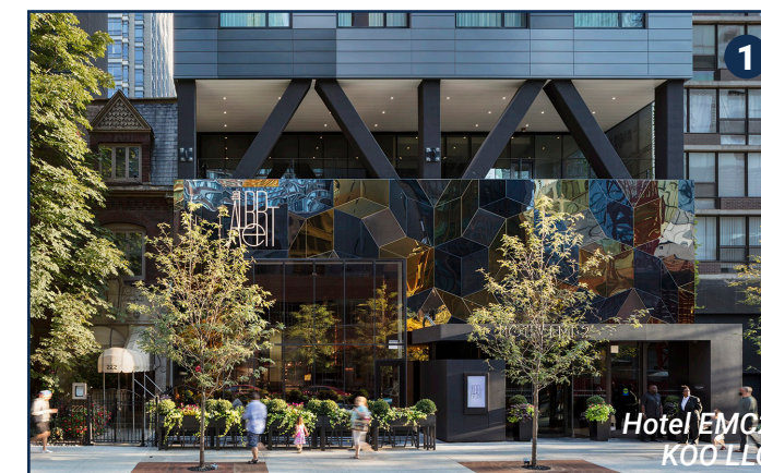
Stainless steel in three colors are used to create a colorful, sculptural, and inviting entrance.
