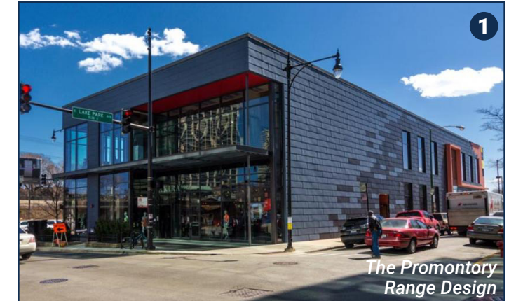
Adding a bar and event space created social activities and nightlife in a commercial corridor lacking those amenities.
