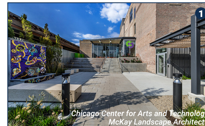
Enlarged entry plazas can be inviting both to building users and the broader public.
