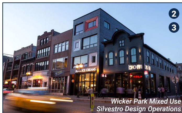
Geometrically interesting window details provide depth and visual interest along the street wall.
