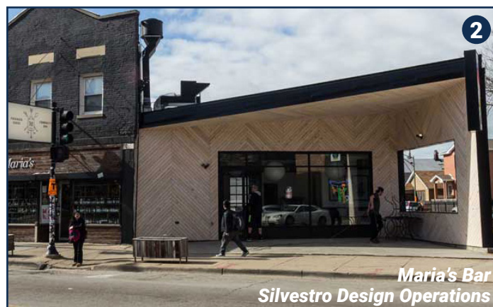
Broadway Streetscape Uptown Transystems and Altamanu Complete street system with generous pedestrian space, plantings, site furniture, and public art
