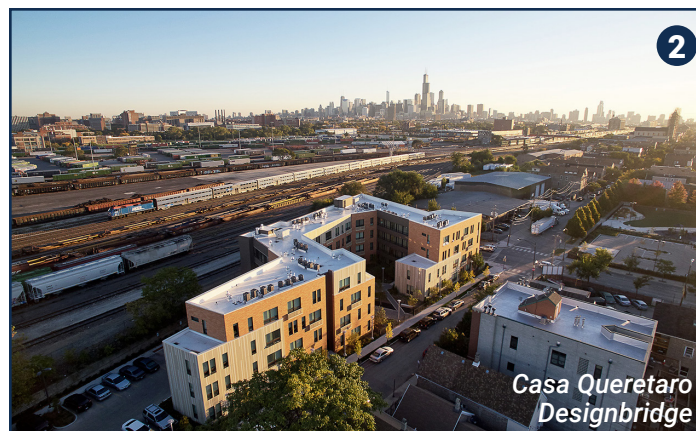
A single-loaded corridor along the adjacent railroad shields residents from noise and provides views of the courtyard.
