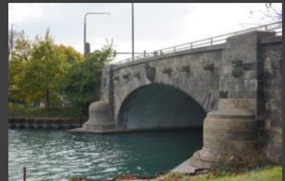
South Haven Bridge (Animal Bridge); 1904
