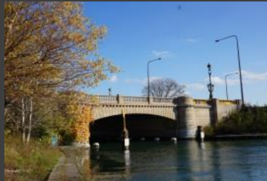
59 th Street Inlet Bridge; 1895
