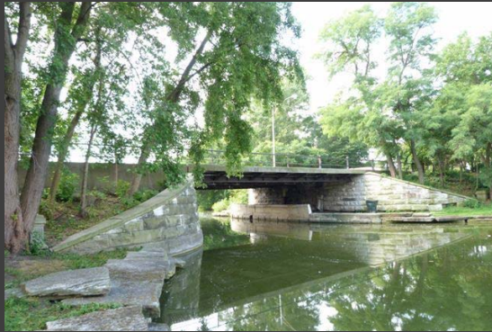
C. Darrow Bridge; 1880; 1893-5; 1957-63
