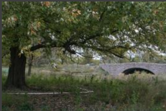
Hayes Drive Lagoon Bridge; 1901
