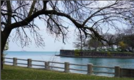
Historic Walls + Balustrades
