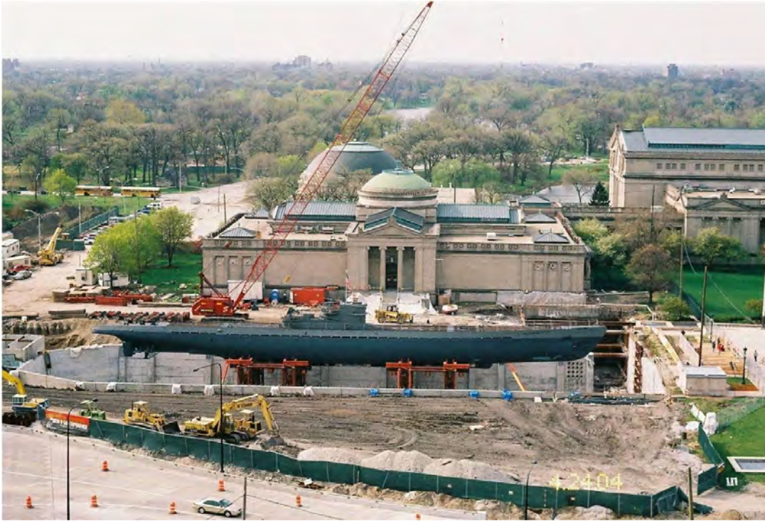
Figure 3.12. Ca. 2009, construction of the underground vault for the U505 submarine immediately north of the Museum of Science and Industry (Jones, Lang Lasalle IP, Inc. 2017).
