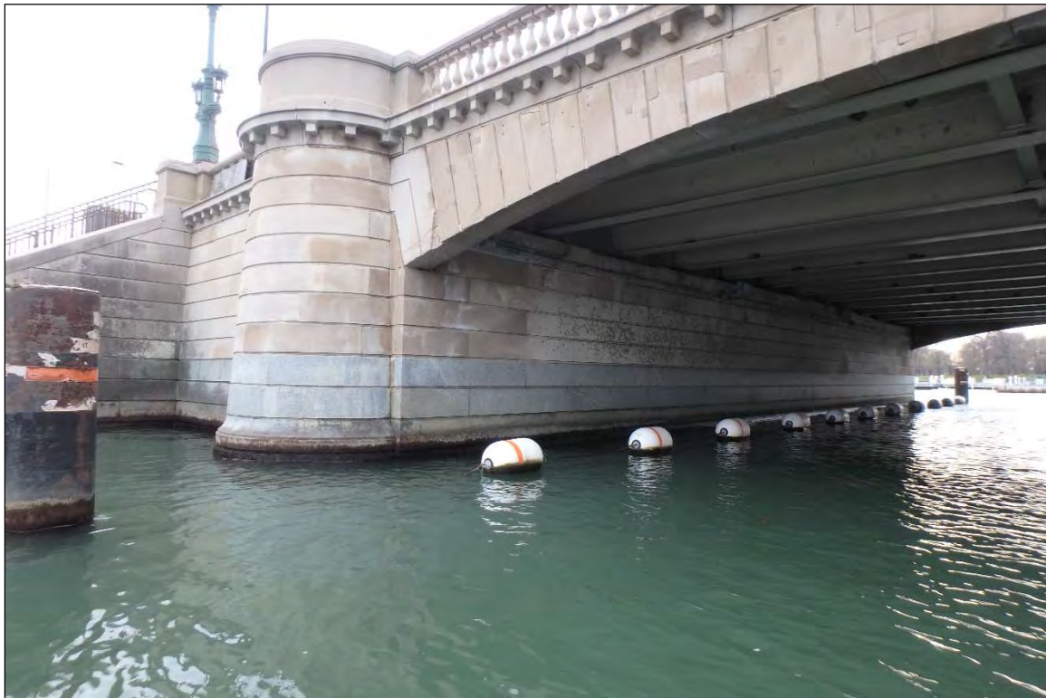
Photographs 4: View of the South River Pier, Looking Southwest.
