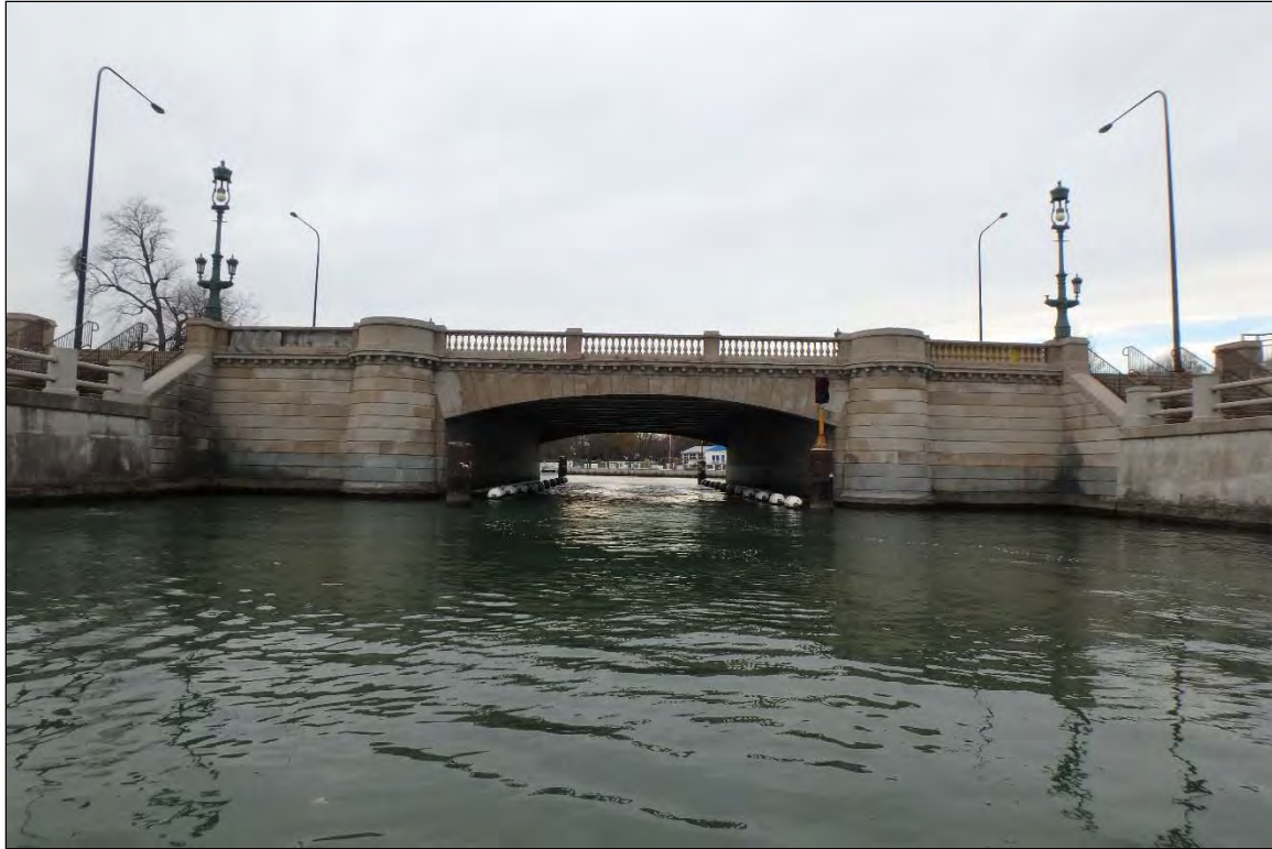
Photographs 1: Overall View of Structure No. 016-6195, Looking West.
