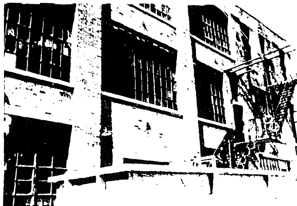
6. Rear of Building No. 4.
