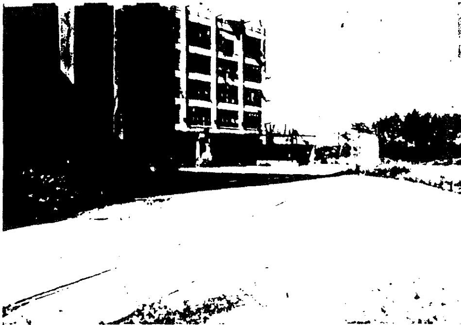
5. Rear of Building No. 6, 7 and 8 and rear service yard.
