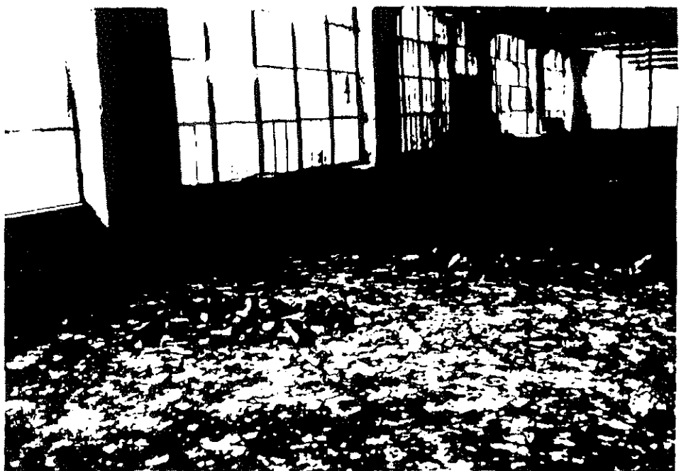
24. East side second floor of Building No. 9.
