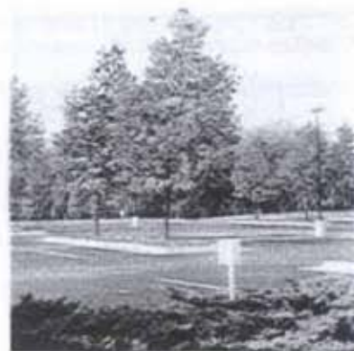
Internal islands of parking lots should be planted with shade trees and groundcover to improve the aesthetic quality of the lot while reducing heat and glare from the sun.
