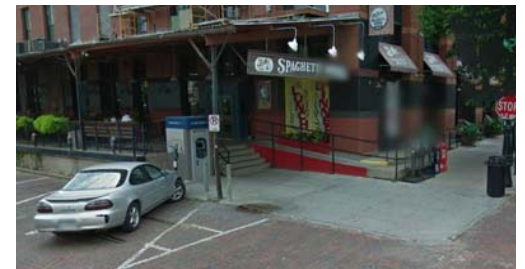
Strong example of a cohesive entry experience integrating ramps and stairs from sidewalk level
