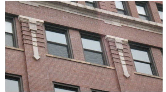
Historic brick masonry with limestone detailing
