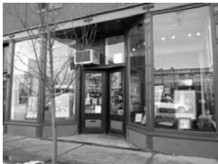
Example of a historic storefront
