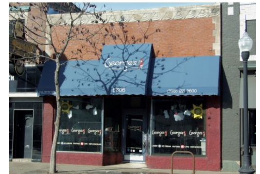
Inappropriate design. Awnings should not cover ornament or other character defining building features
