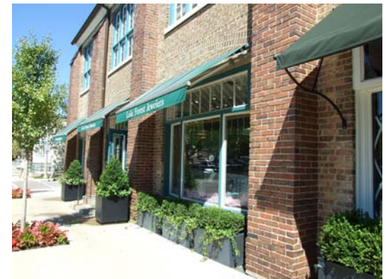
Example of appropriate awning design showing shed type awnings located over individual storefronts.
