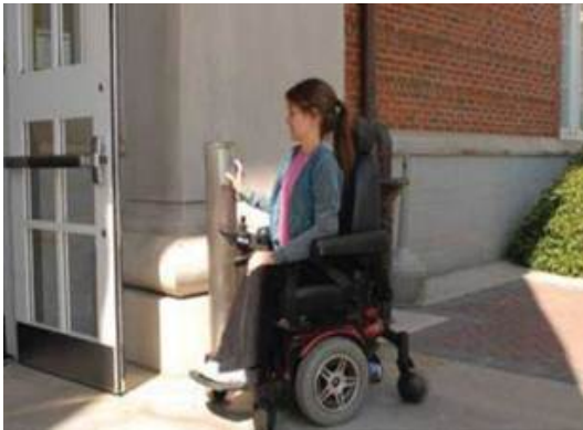
Push plate to operate automatic door opener
