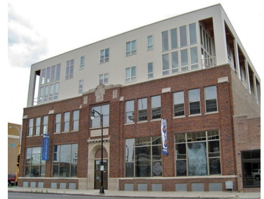
Example of poorly designed rooftop addition.
