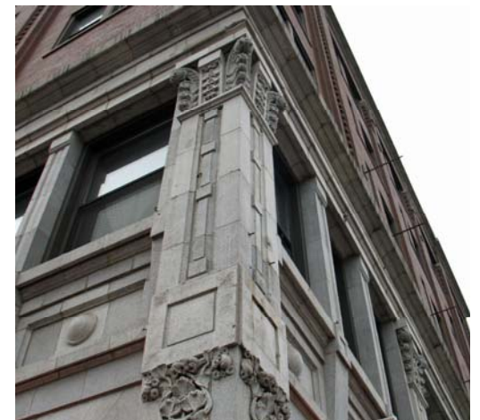
Historic terra cotta at base of building.
