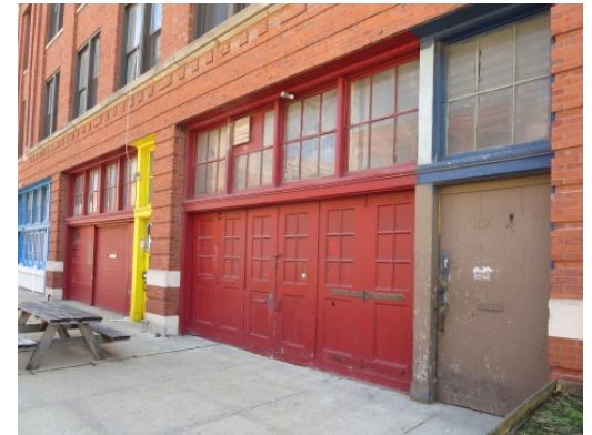
Historic industrial doors at Fulton Market
