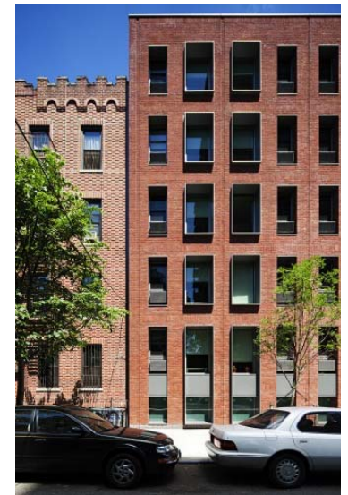
Appropriate new construction
