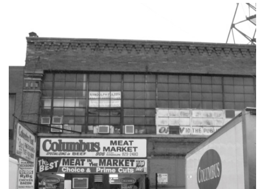
Historic steel windows on Randolph Street
