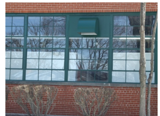
Appropriate new steel windows
