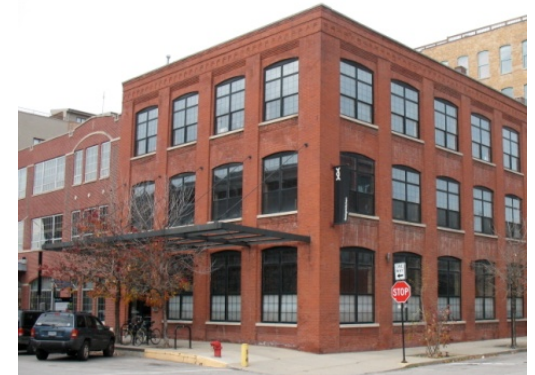
Existing historic canopy frame at Fulton Market
