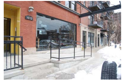
Strong example of creative ADA compliance ramping and railing design along the side street
