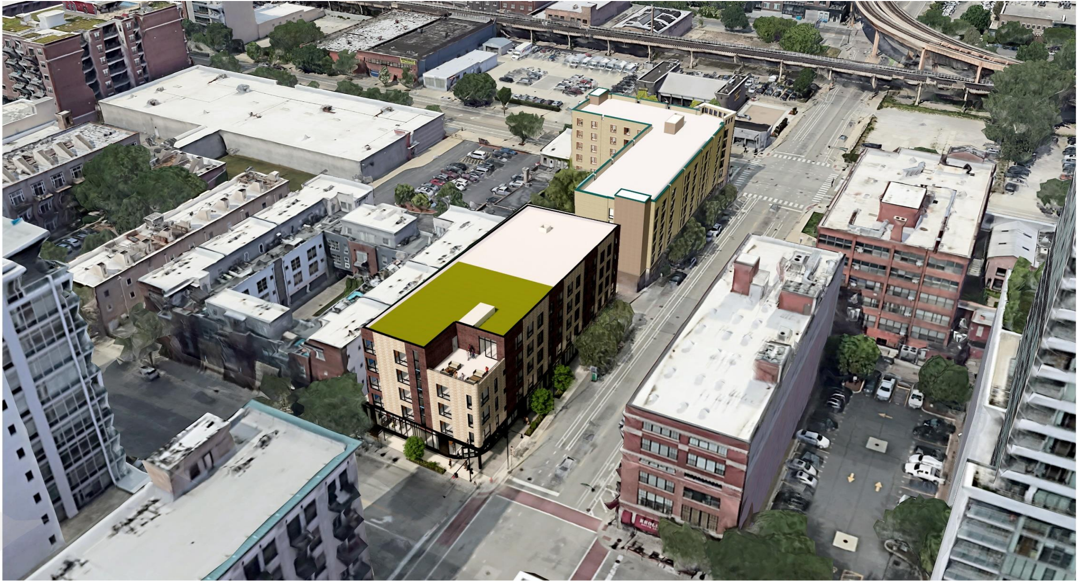
NORTH EAST AERIAL VIEW
